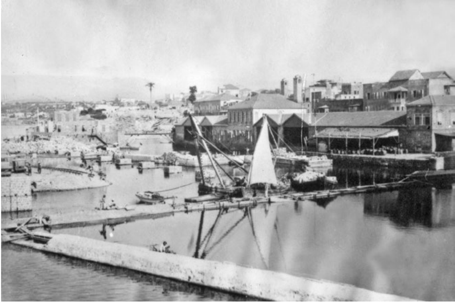
14. Yıldız Fotoğraf Koleksiyonu, 90662/20: A view of the construction work on the mole of the port of Beirut, July 1892.
