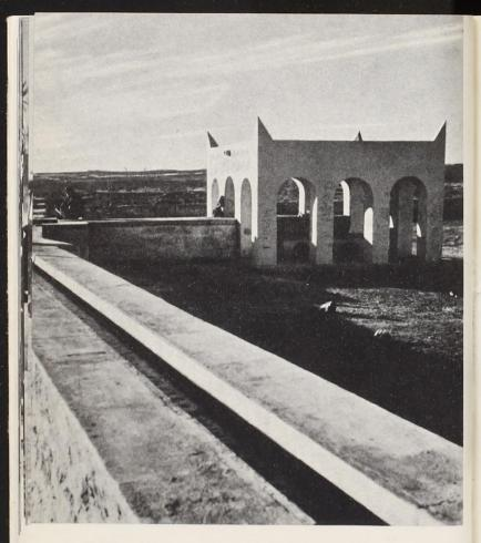
From the spring's reservoir near Brak in the Wadi esc Sciati artesian water flows through masonry troughs into the gardens.
