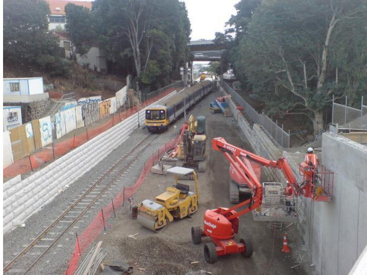
Fig. 8.2: Construction work slowing regular speed on a track. Image [Cc0a]
