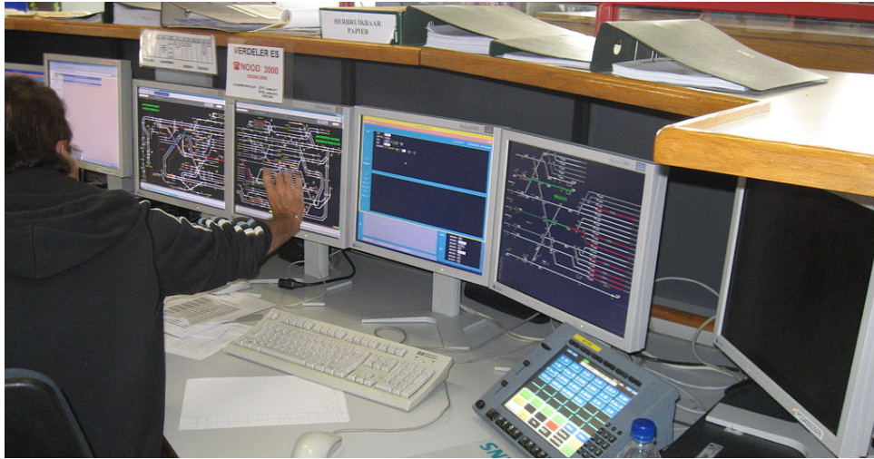
Fig. 4.1: Workplace of dispatcher[Com07]. The hand of the dispatcher points to a monitor displaying track allocation.
