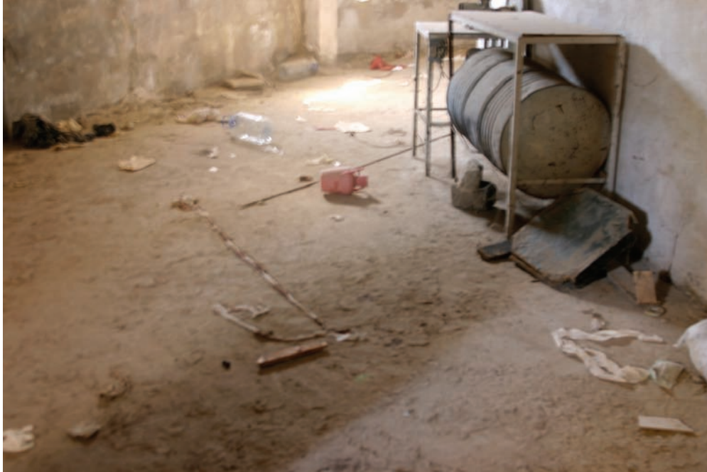
The Qana basement in which the wounded ambulance crews and Muhammad Fawaz took shelter. The floor of the basement was still littered with discarded first aid equipment when visited by Human Rights Watch on September 14. © 2006 Peter Bouckaert/Human Rights Watch
