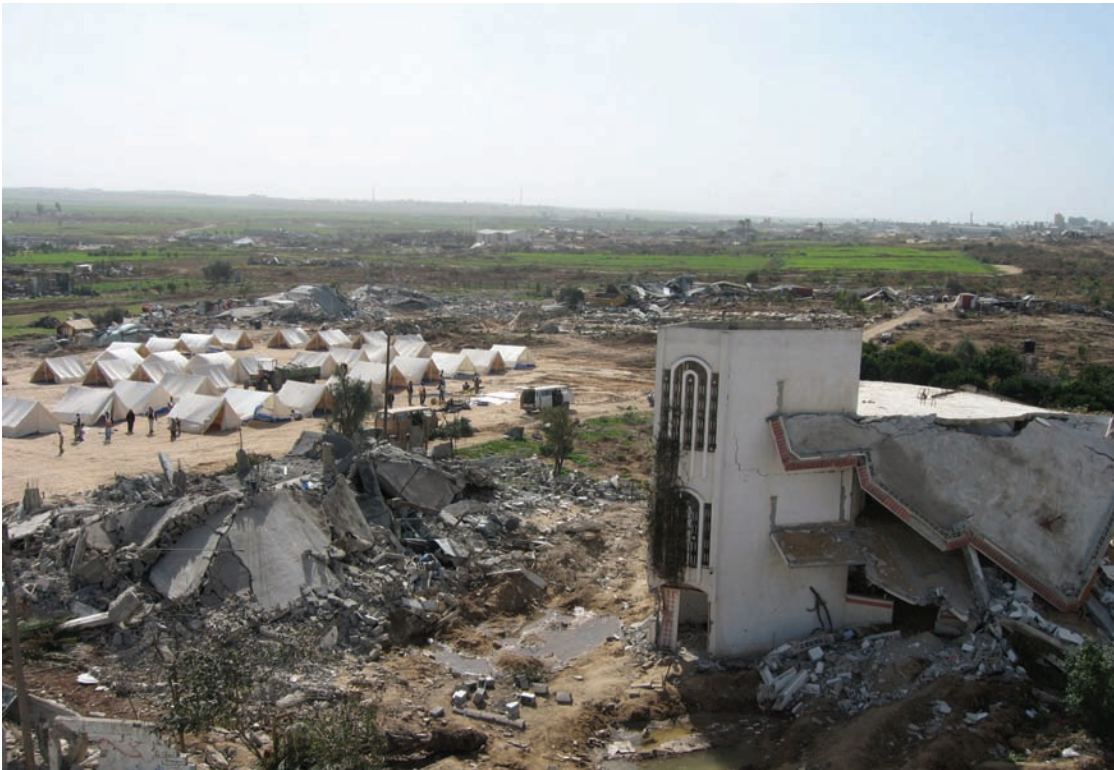
Destroyed buildings and a tent camp in Izbt Abd Rabbo, April 2009. Human Rights Watch documented the complete destruction of the homes of at least 287 people on or near the neighborhood's main road. © 2009 Bill Van Esveld/Human Rights Watch.
