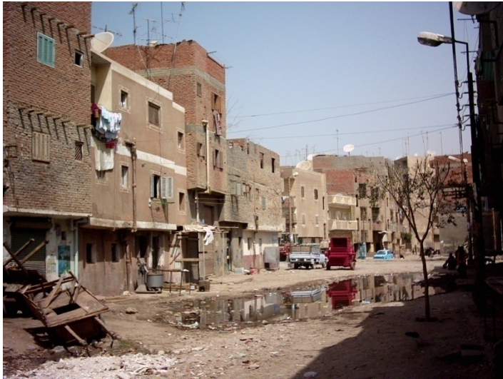
Figure 2-4 Example of an informal settlement lacking infrastructure
