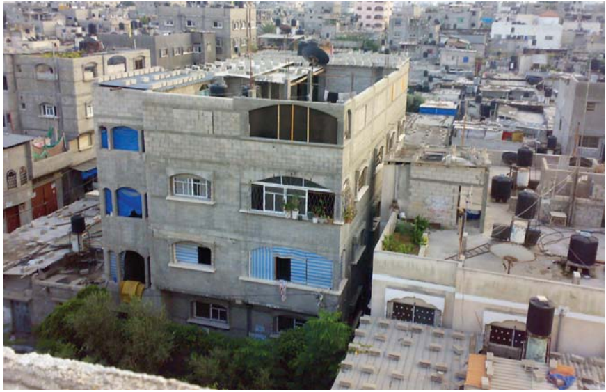
Figure1.13 Jabalia refugee camp, most of the houses are permanent
