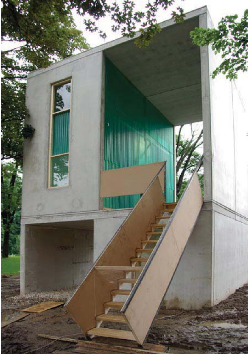
Figure 2.11 Mock-up of the unit
