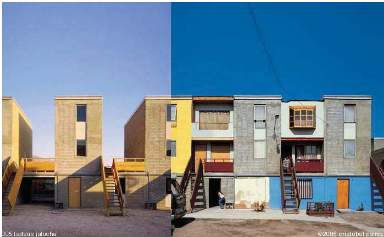
Figure 2.6 The controlled expansion of Quinta Monroy housing project, the photo on the right was taken a year after the project was completed
