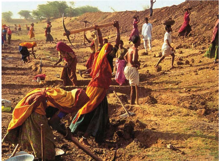
Figure 3.8 Residents are involved in construction in the Barefoot projects
