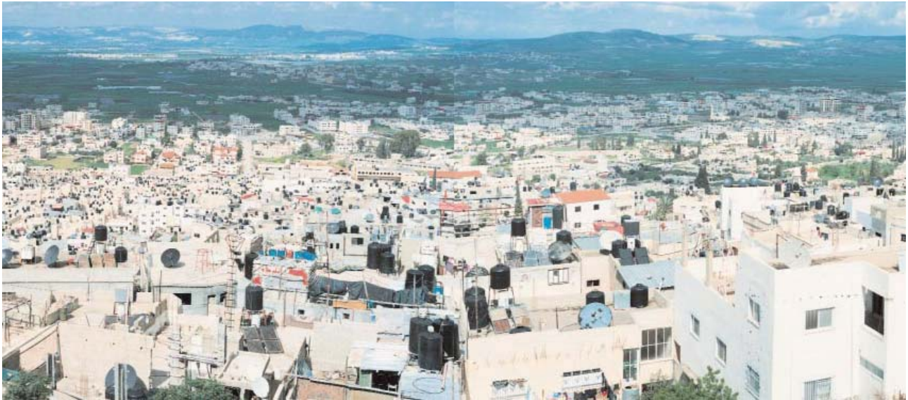
Figure 4.7 Jenin camp after reconstruction
