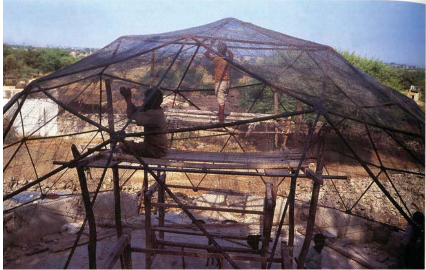
Figure3.11 using metal scraps to build the dome
