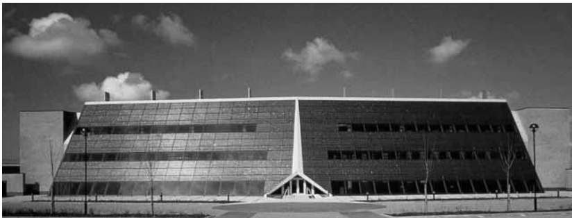
Fig. 4-37 : Solar Office, Doxford International Business Park, facade.
