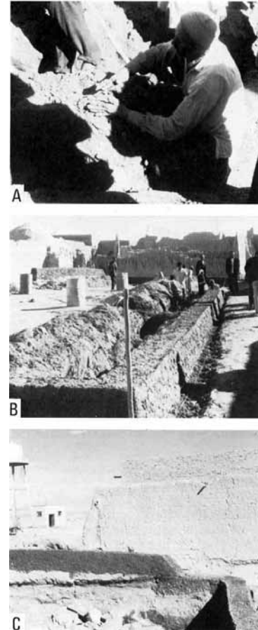
Fig. 1-23: Puddled mud walls, Iran. A) Mud is shaped by hand without use of forms. B) Mixing is done on the ground adjacent to where the mixture will be placed. A corner pole and line is used to maintain direction and level. C) Build-up to the wall is done in sequence, allowing earlier courses to dry. In the background, note difference between brick wall and puddled mud wall.
