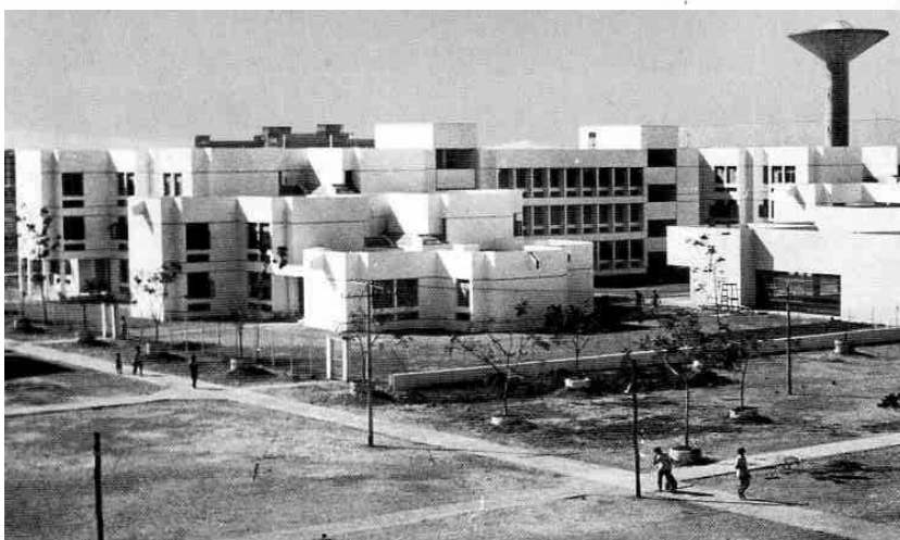
Fig. 1-42: C.M. Correa & et al (India): typical image of the public housing in developing countries at the end of 60s and 70s.
