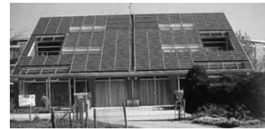
Fig. 4-27: Residential buildings, the double residence new housing district, Nieuwland.
