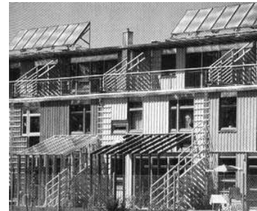
Fig. 3-7: Simple collectors of the “flat plate” type; Apartment building, Germany.
