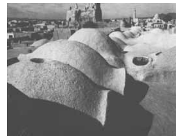
Fig. 1-24: The roof form helps to reduce the effect of heat and wind in arid regions.
