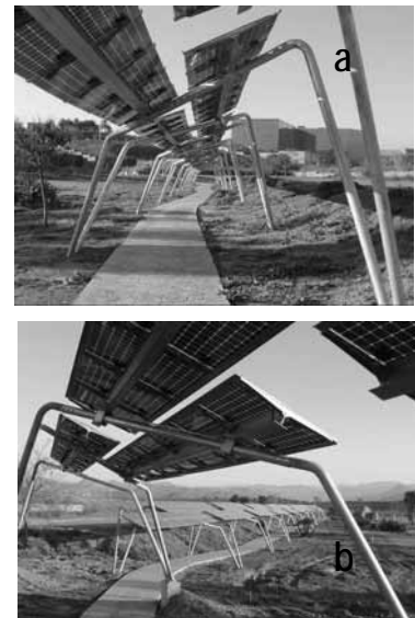
Fig. 4-41 a&b: Photovoltaic pergola installed in the Andalusia Technology Park in Malaga
