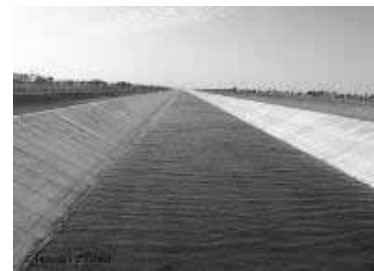
Fig. 6-16: Sheikh Zayed Canal
