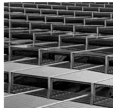
Fig. 4-33: Mont-Cenis Academy, Germany, the PV roofing detail.
