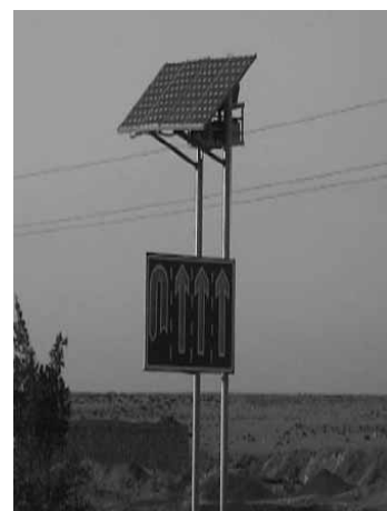
Fig. 6-6: Egypt, Using PV for street lighting and for signs.
