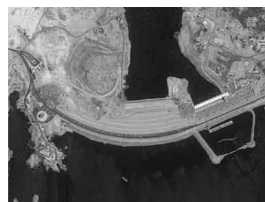
Fig. 6-3: The High Dam, Aswan. One of the main sources of energy in Egypt.
