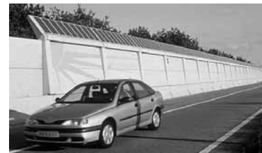
Fig. 4-44: PV noise barrier A27. Netherlands.
