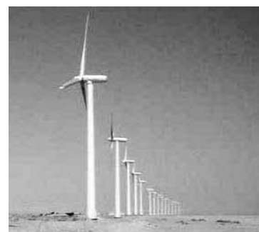
Fig. 6-2: 225 MW wind farm at Zafarana:
