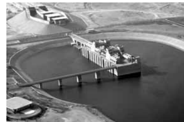
Fig. 6-15: Mubarak Pumping Station
