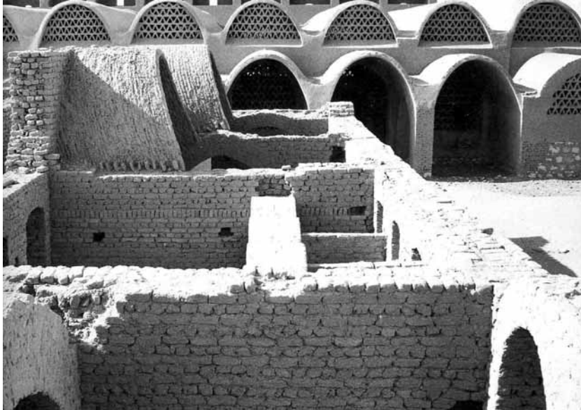
Fig. 1-38: Using the traditional materials with the traditional forms. New Bariz, Egypt: the village's market.
