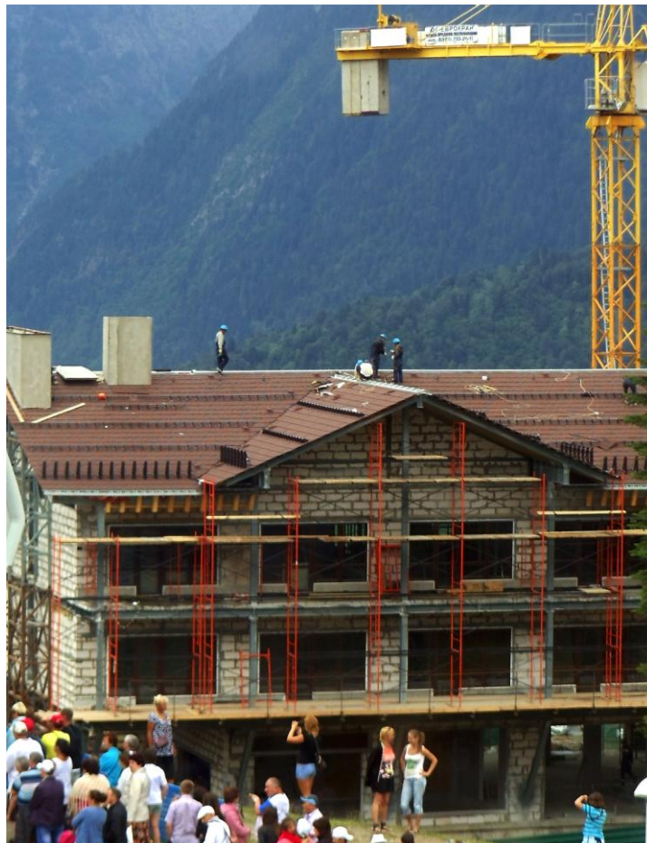
Working on Roof (Rut Perez-Studer, Olympic construction site, Russia, 2012)
