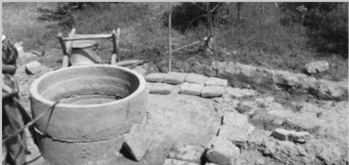
Figure 15: Dug well on a farm to supplement canal irrigation
