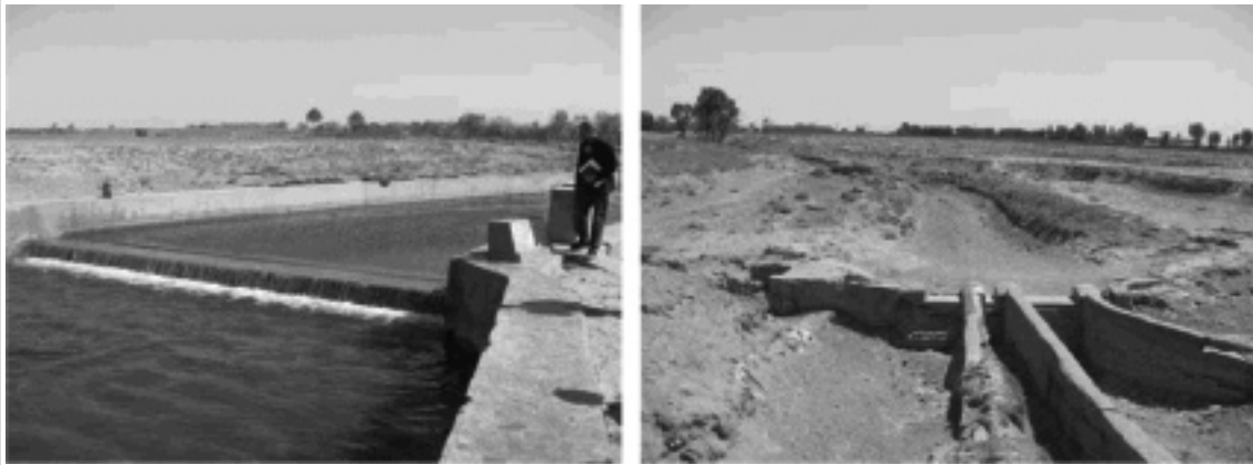
Figure 11: Flows in the upper section (close to Herat) and lower section (Ghaibatun village) of the Injil canal
