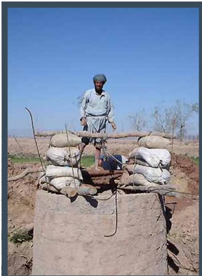
Illustration 18: Well construction traditional method (Bob Rout photograph)
