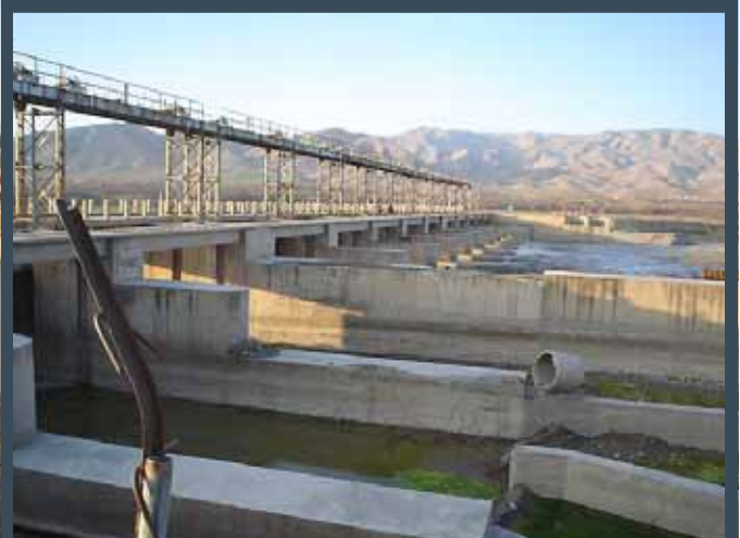
Illustration 21: Diversion weir, Kunduz-Khanabad (Bob Rout photograph)
