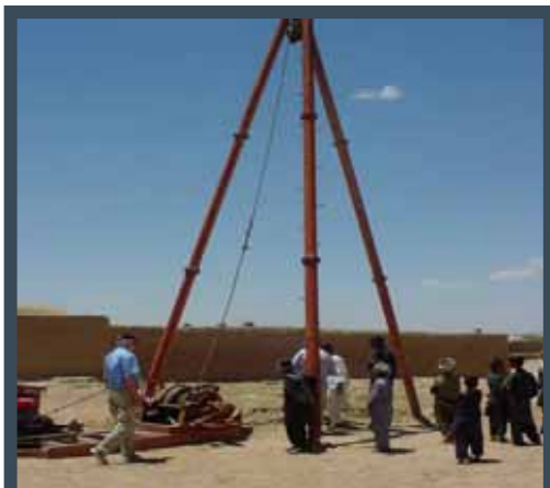
Illustration 19: Modern well-drilling (Bob Rout photograph)
