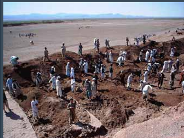
Illustration 1: Annual maintenance on Joy Naw main canal, Herat (Bob Rout photograph)
