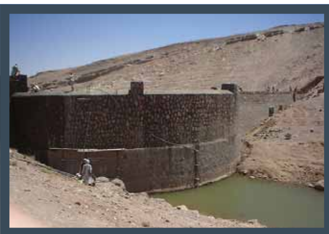
Illustration 13: Dam under construction
