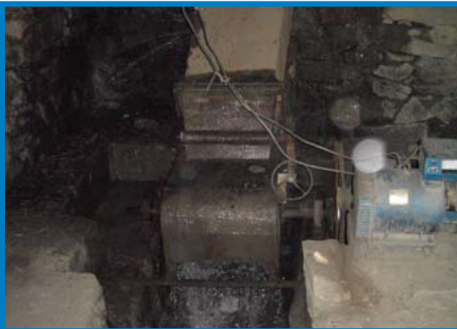
Photo 20. Pacha Joi Canal, Laghman Province
