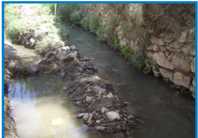
Photo 7. Kama Canal, Nangarhar Province
