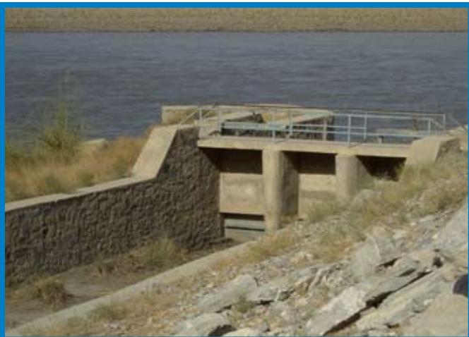
Photo 26. Kama Canal, Nangarhar Province
