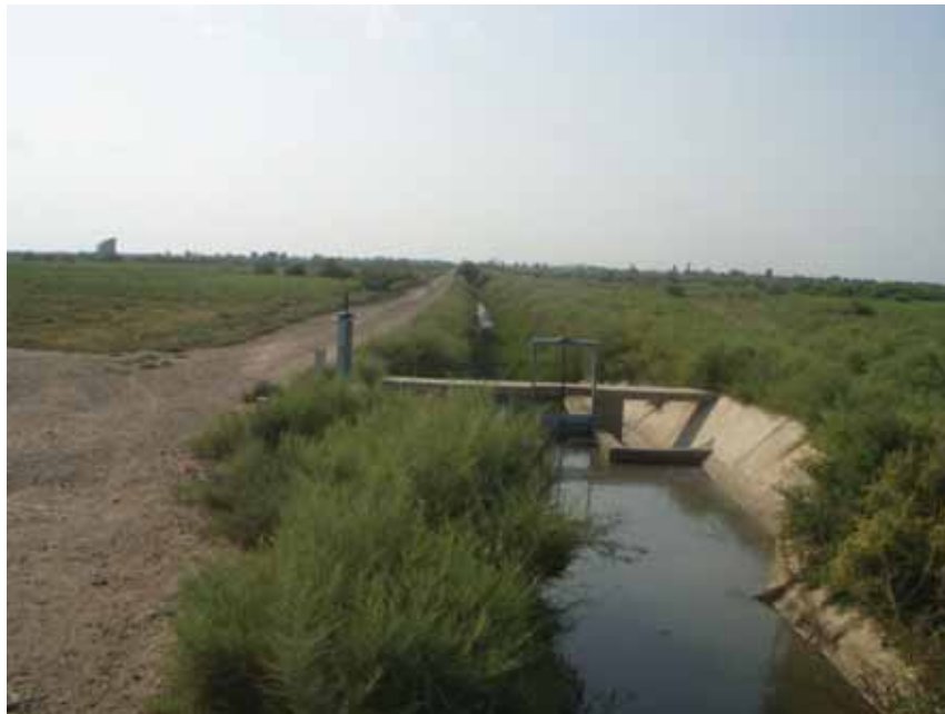
Photograph 4 : Rehabilitated canal in Jaferli WUA, Imisli (August 2011)
