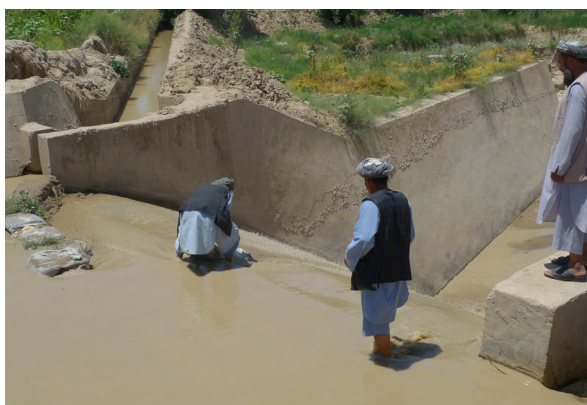
Image 16: A canal mirab removes sandbags from a proportional divider, Jawzjan Province.
