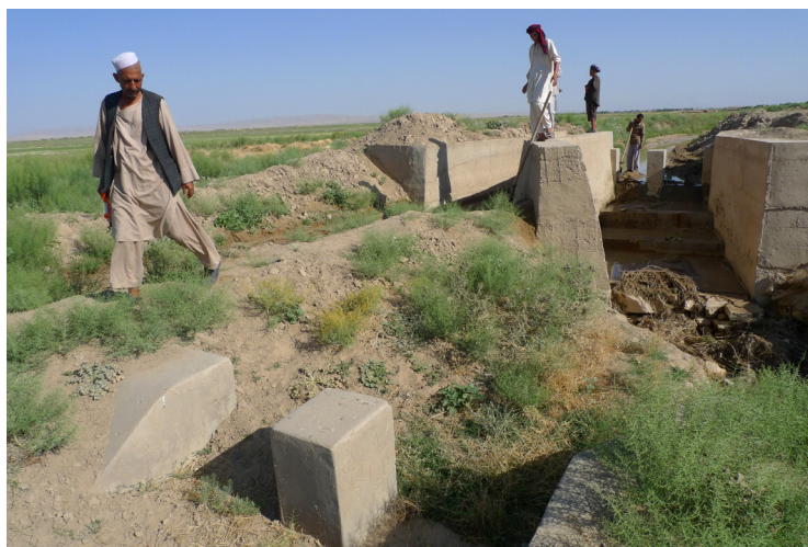
Image 19: Old structure (foreground) and new structure (background) of Emshek / Altkhoja
