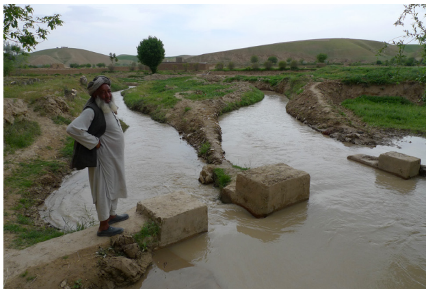
Image 21: Afredi Divider. Left branch supplies the land around Afredi village; right branch supplies the main canal going toward Akhtash and other villages.
