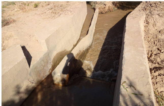
Image 18: Jui Qawchin (left) and Nahr-i-Salmazan (right) following the PC head's decision. Note that the original NGO construction (left) has been filled with cement.
