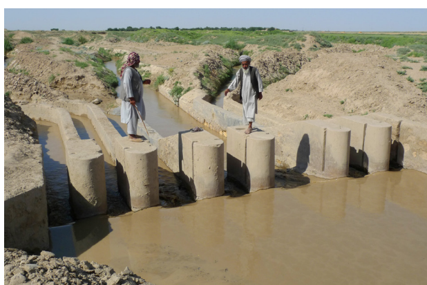
Image 8: Proportional divider with six branches (shash darak; note that the fourth branch (from left) has two openings to make it easier when branches have to be closed for maintenance).
