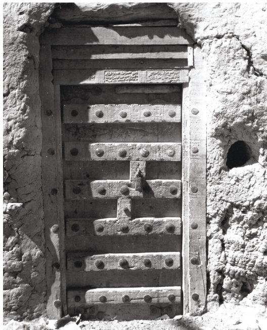
Figure 62. al-Hajarayn. An entrance door: in the centre, the door hammer; below the lintel, the carpenter's inscription; to the right, a hole in the wall for opening the latch.
