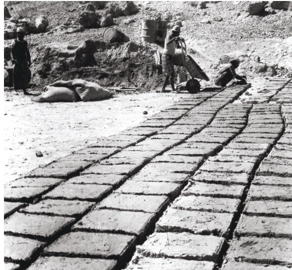
Figure 69. Making mud bricks.
