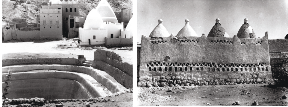
Figures 73–74. Mashhad ‘Alī, Wādī Daw‘an: irrigation reservoir ( jābiyah ); to the right a cistern of drinking water ( siqāyah ).
