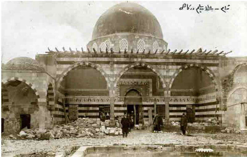
FIGURE 9.6 The Madrasa al-Salimiyya during the renovation: Damascus – The dervish lodge of Sultan Selim (Şâm – Sulţân Selîm dergâhı). Courtesy of Wolf-Dieter Lemke, Berlin.
