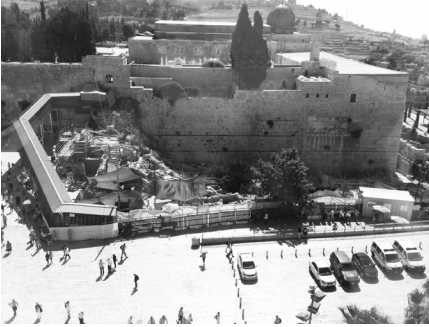
FIGURE 39. Mughrabi Gate ramp and excavations. Photo by Katharina Galor.
