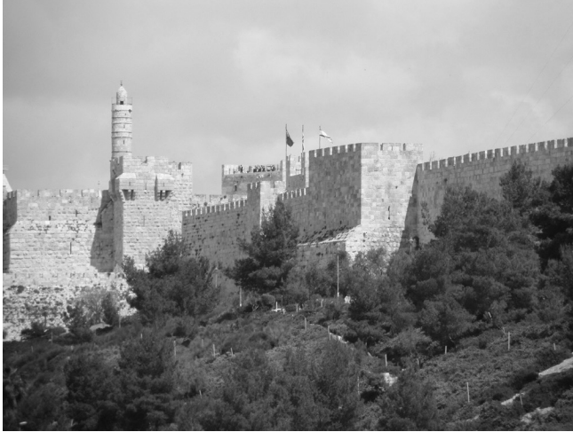
FIGURE 2. Section of Ottoman city wall, south of the Citadel. Photo by Katharina Galor.
