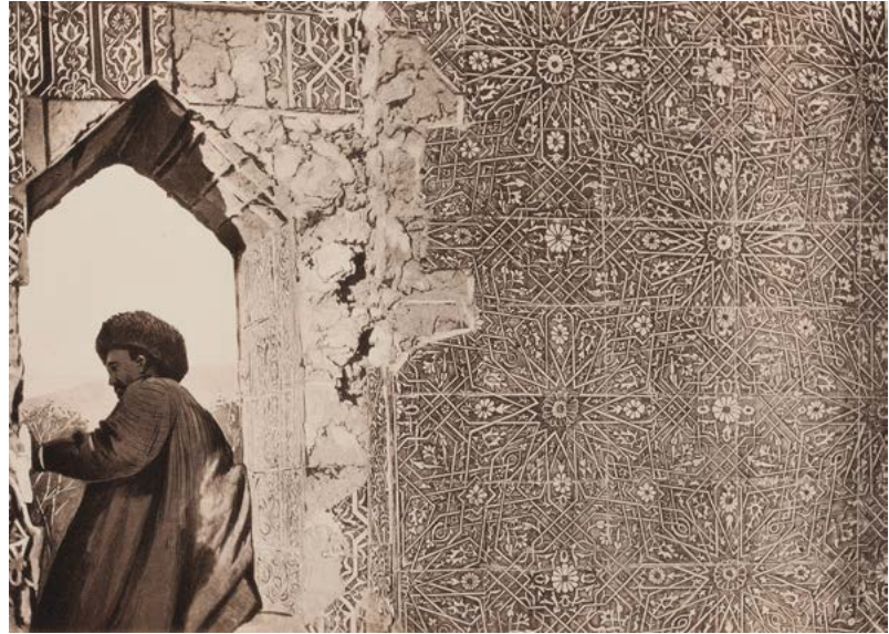
Figure 15: Here a local in Khiva is photographed removing tiles from a mosque to fulfil an order for a collector. Source: d’Allemagne, 1911.
