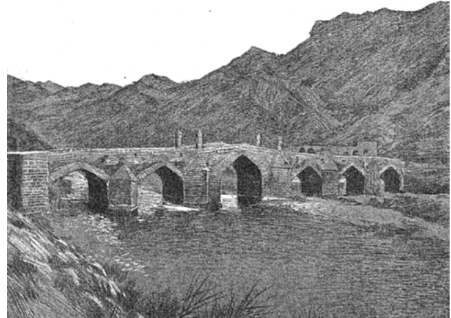
Figure 29: The bridge at Daliki. Vilmorin (1895).
