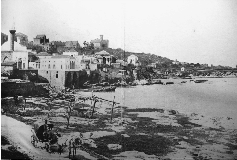
Fig. 2: View of Ras Beirut, late 19 th century. Source: Bonfils photograph in Bayard Dodge, The American University of Beirut; A Brief History of the University and the lands which it serves (Beirut: Khayat's, 1958).
