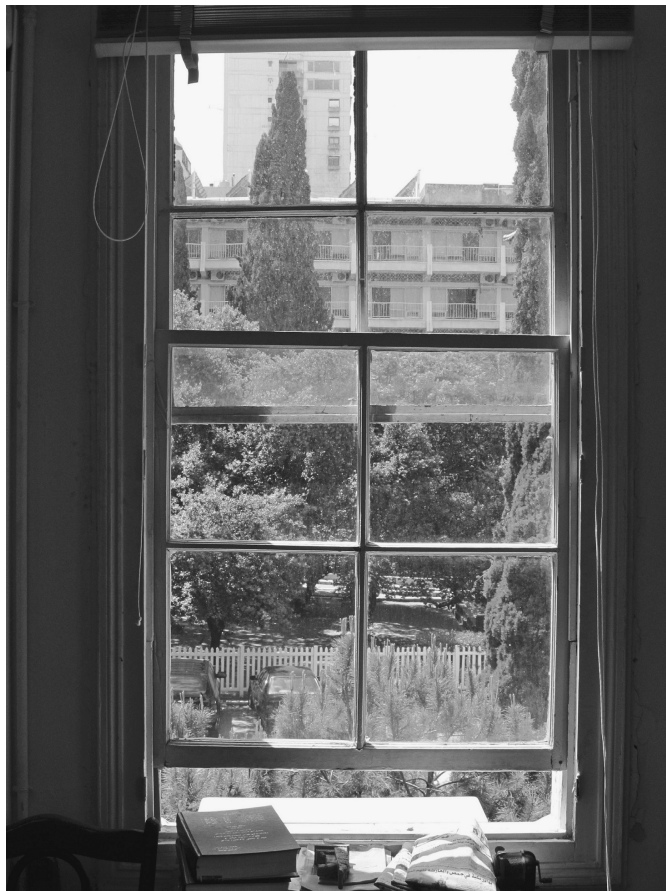
Fig. 1: Double sash window, Fisk Hall, American University of Beirut. Source: Photograph taken by author.
