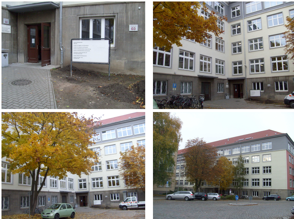
Figure 4.10: Outside views of building 2 and 3 used for recording the data
