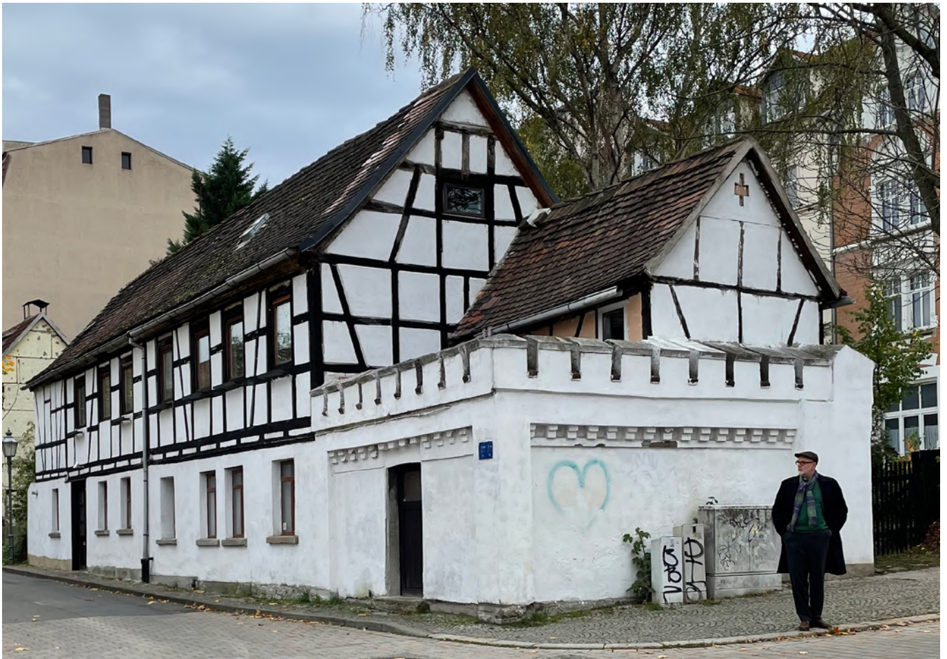
Figure 17: Photograph of surrounding buildings. By author.
