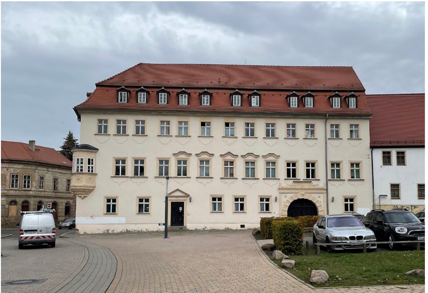
Figure 16: Photograph of surrounding buildings. By author.
