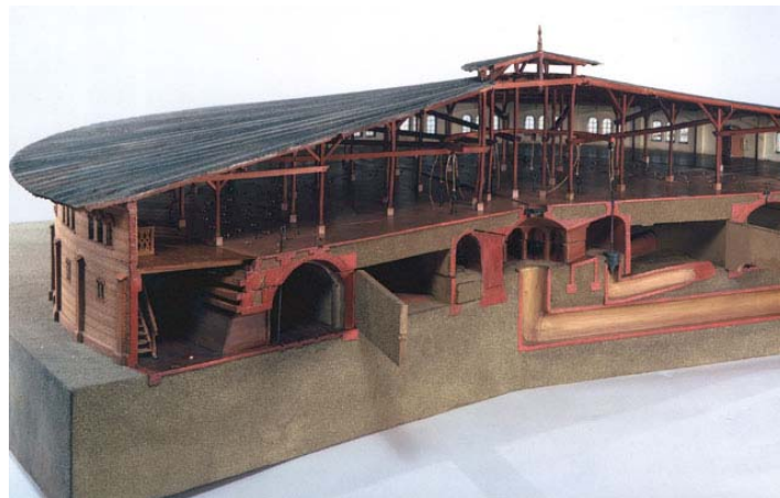
Figure 1.7: Scale model of Hoffmann kiln [7]
