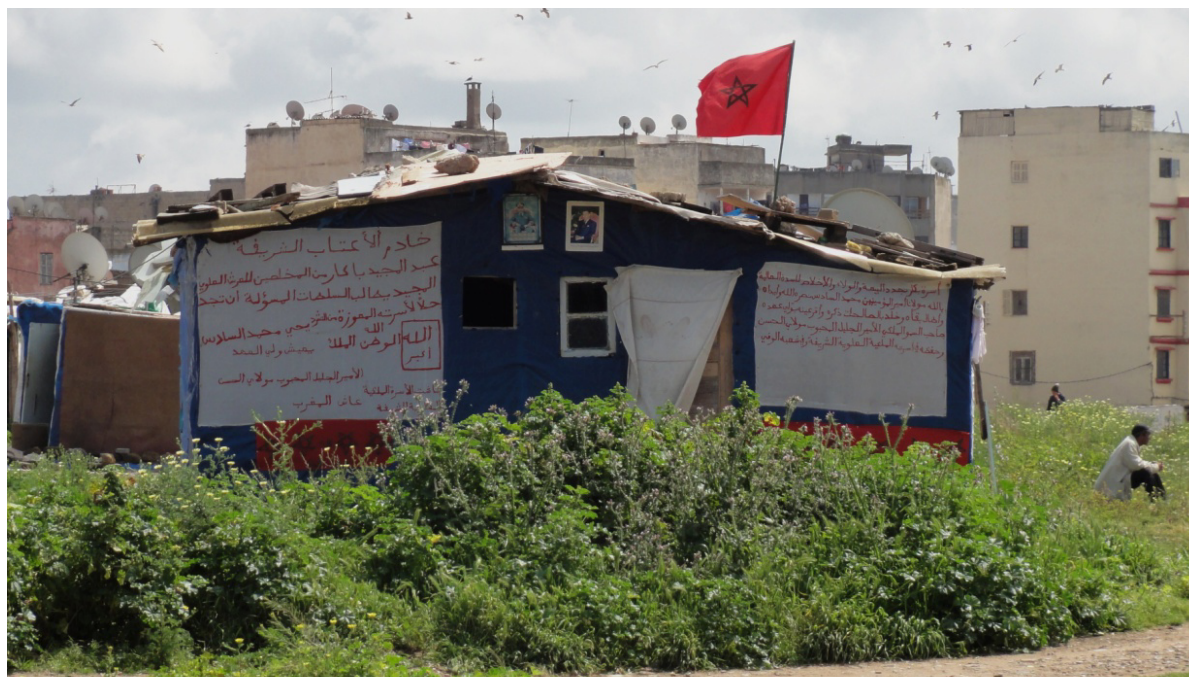
Figure 7: A royalist house owner protests against his eviction caused by the construction of the Royal Avenue in the medina of Casablanca
