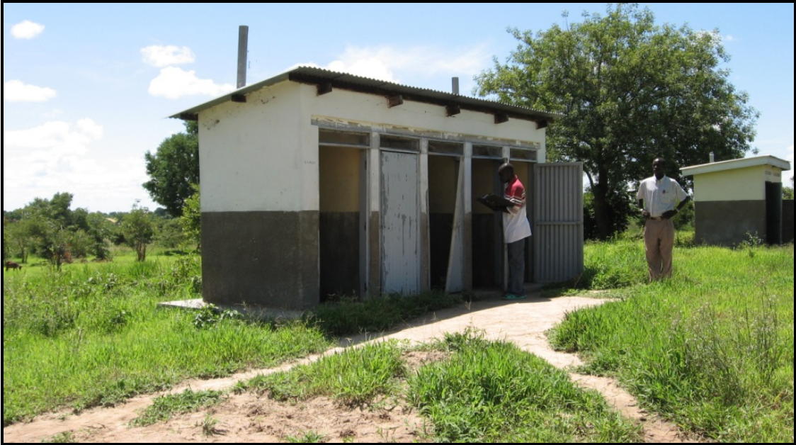
Figure 13. Pit Latrine, 5 stances.
