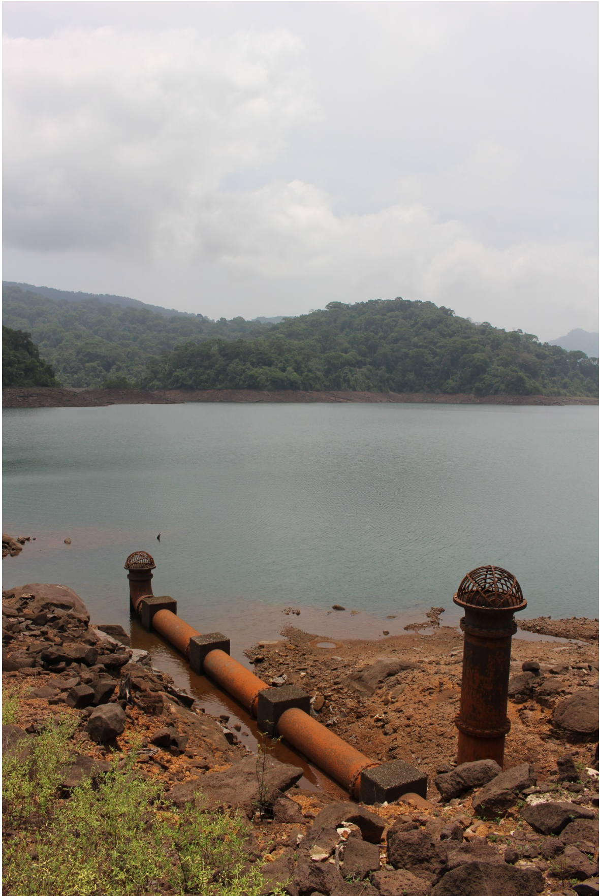
Figure 2.1.: The Guma Dam and two of its intakes during dry season (photo taken by Lorenz Gosch)
