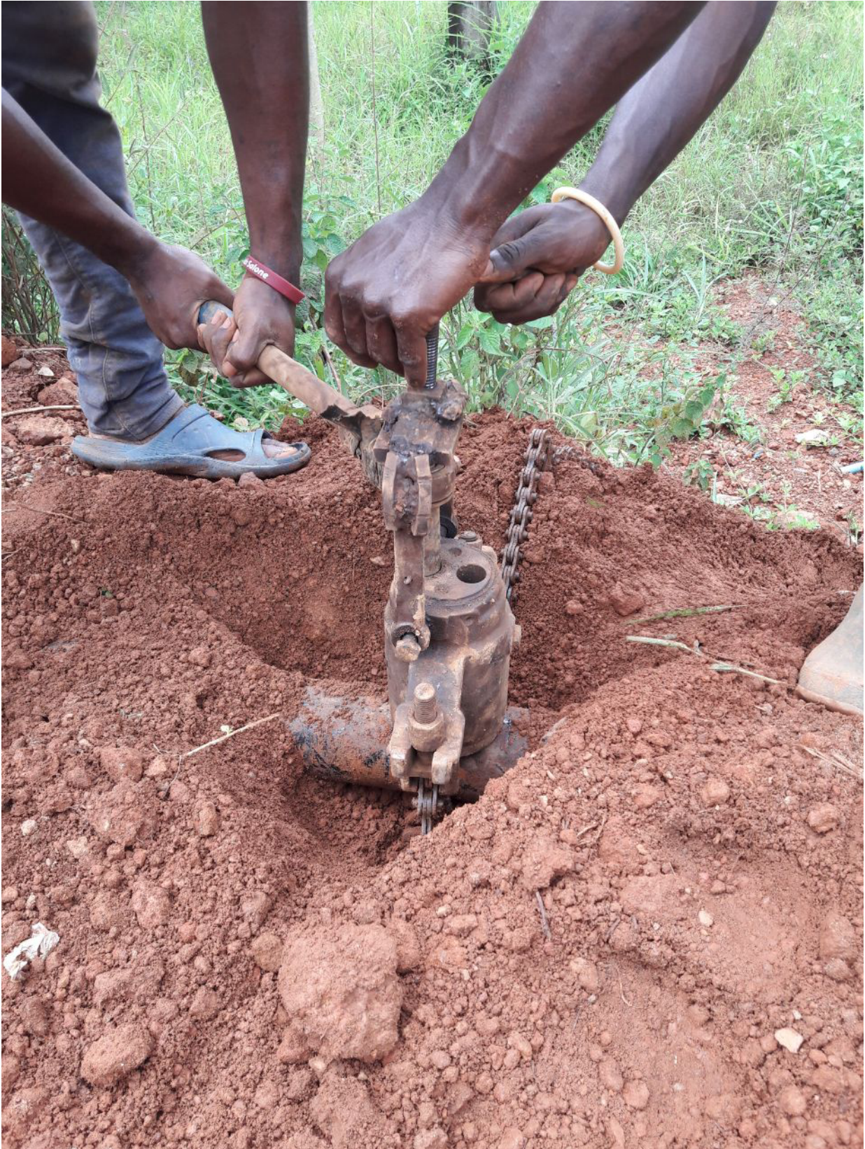
Figure 4.3.: Putting the drill to work: Making a connection on a sub-main (photo taken by Lorenz Gosch)
