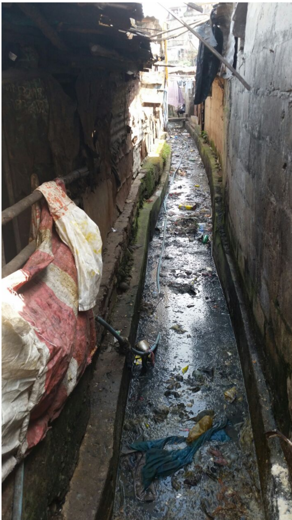
Figure 5.3.: Pipe in the gutter (photo taken by Lorenz Gosch)
