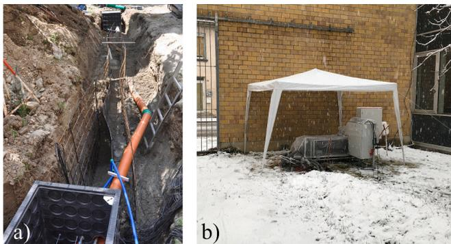
Fig. 5. a) Trench collector and measurement equipment during installation, b) thermal response test device attached to the trench collector plant at the experimental site.
