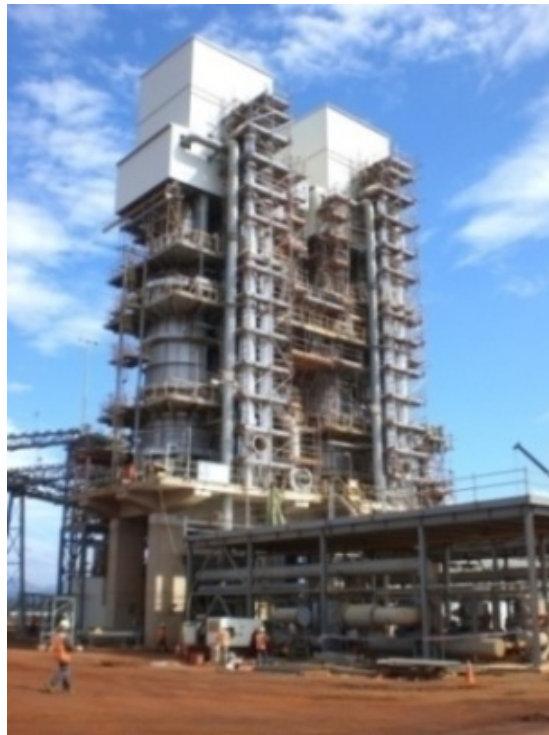
Figure 1-8: PFR- kiln (source: http:// www.cimprogetti.com )
