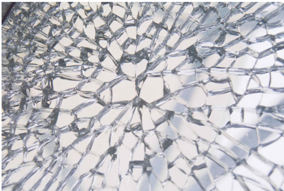
Figure 24: Typical fracture appearance of tempered glass [131]
