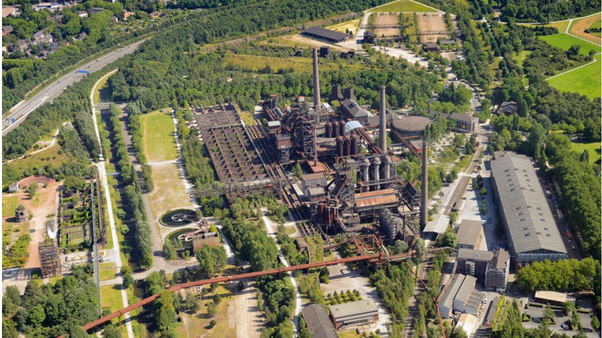
Photo 3: Overview of Landscape Park Duisburg-Nord
