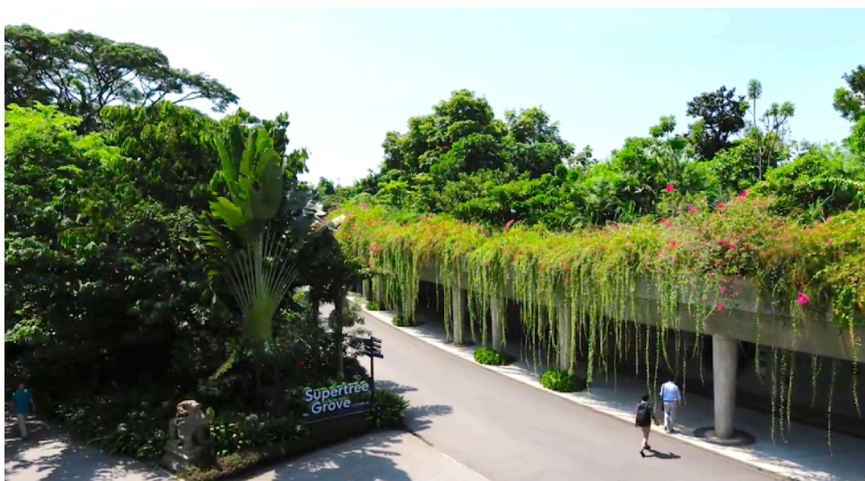
Figure 60- Shows the urban greenery in Singapore ( Green roof).
