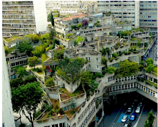
Figure 21- Shows the roof gardens in France.
