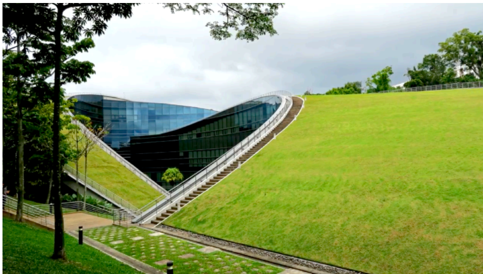
Figure 59- Shows the urban greenery in Singapore ( Green roof).
