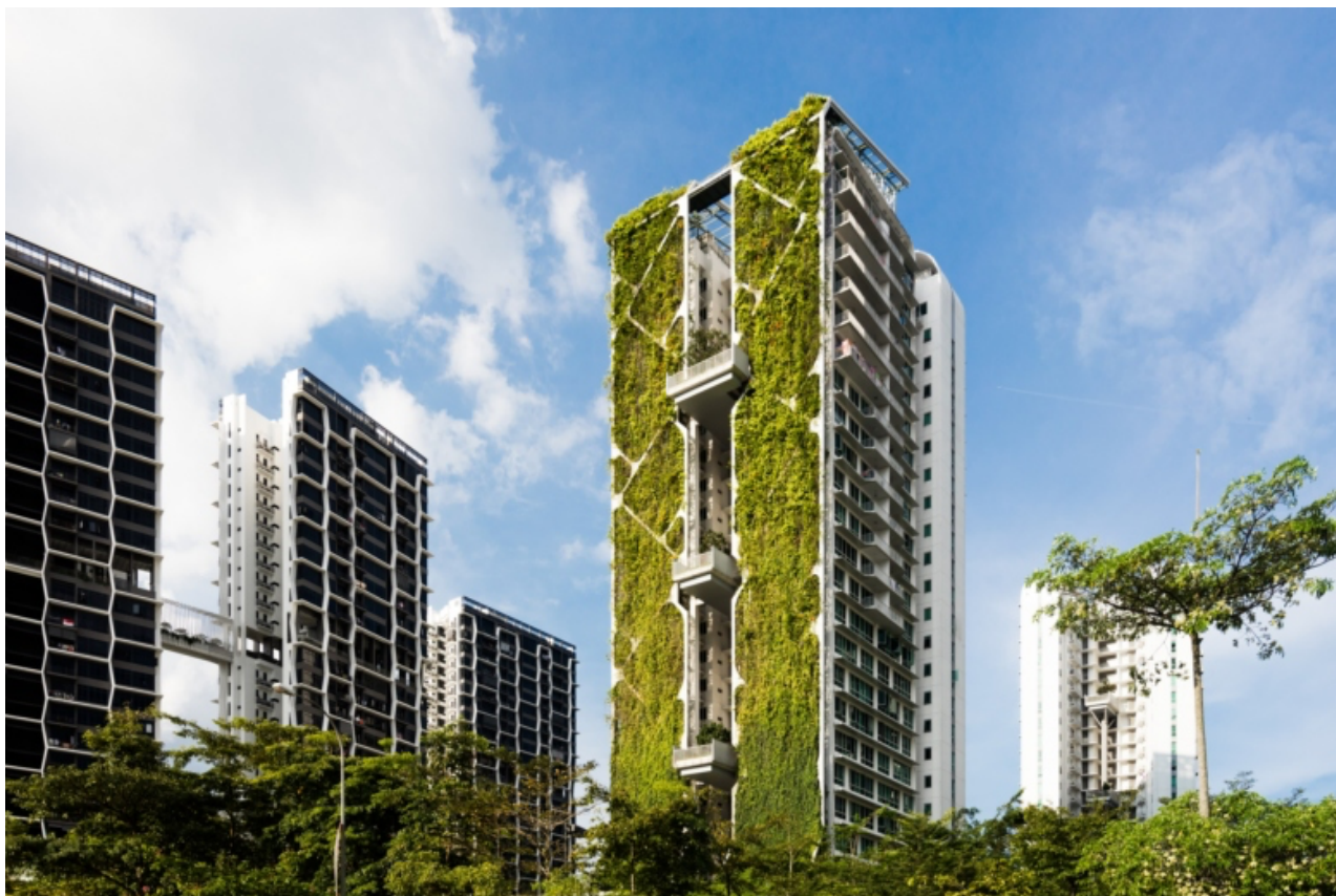
Figure 65- Well designed and maintained green walls on the facade of the tree house, visually impactful and may help reduce the temperature in the vicinity. Source: Finbarr Fallon
