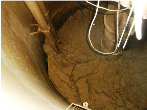
Abb. 0-16 Reaktor verblockt mit 150 m<sup>3</sup> Schlamm
