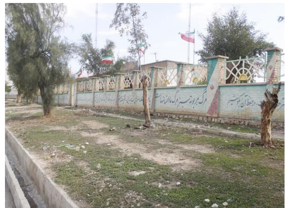
Figure 3.9: Lack of maintenance
