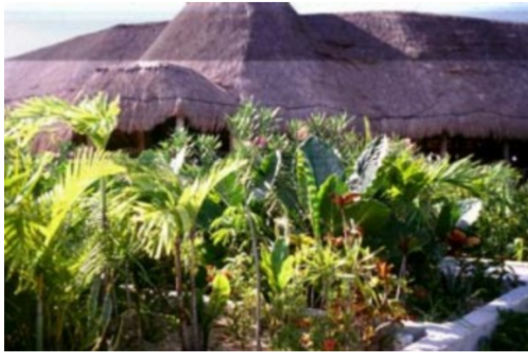
Fig.3.12: Xpu-Ha Eco-Park, Restaurant, handling wastewater for 1500 people
