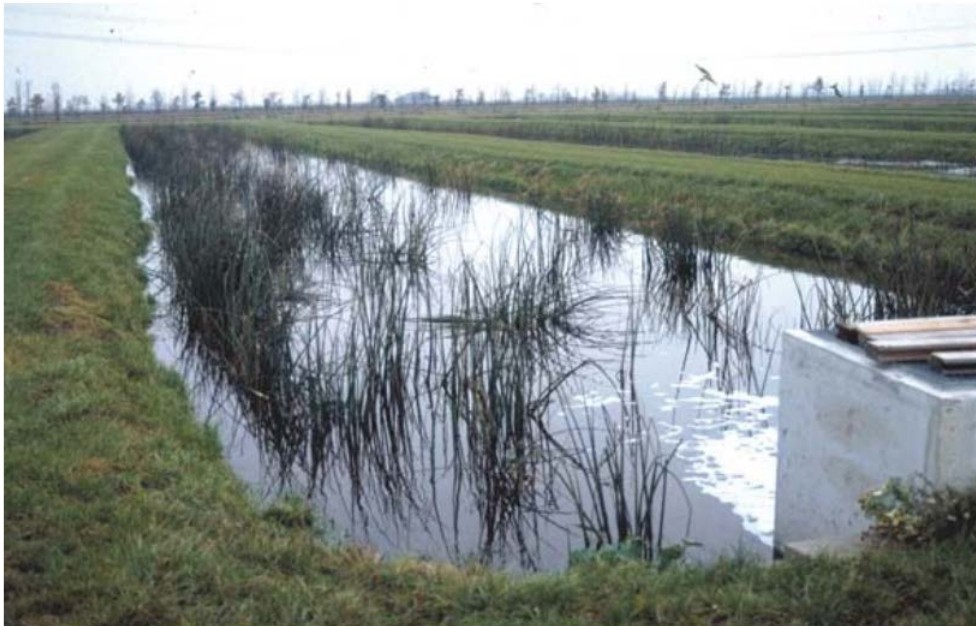
Fig. 3.7: FWS constructed wetland at Leystad, the Netherlands , planted with Scirpuslacustris . Photo by Hans Brix
