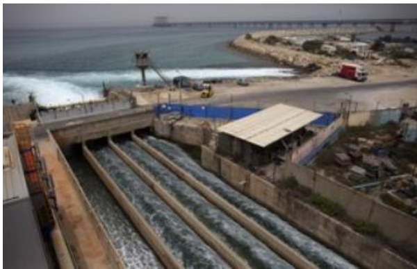
Limassol desalination plant
