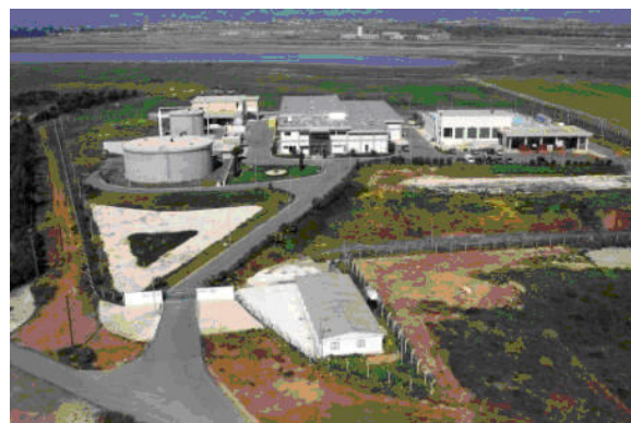
Dhekelia desalination plant
