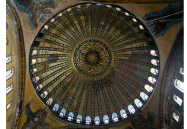
Hagia Sophia in Istanbul was constructed between 532 and 537 CE. The dome measures 55.60 metres over the central space and 31.87 metres from ground level. Because of the repairs and constructions over time, the dome lost its circular shape and the diameter. Photo: Stock-Fotografie-ID:453531275, Gogosvm
