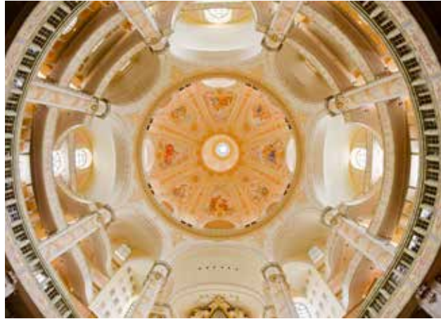
The Frauenkirche, or The Church of Our Lady, was constructed between 1726 and 1743 by the architect George Baehr. Along with the domes of the Florence Cathedral and St Peter's in Rome, this is one of the rare domes to have been built completely in stone. Photo: Stock-Fotografie-ID:471082915, Nikada
