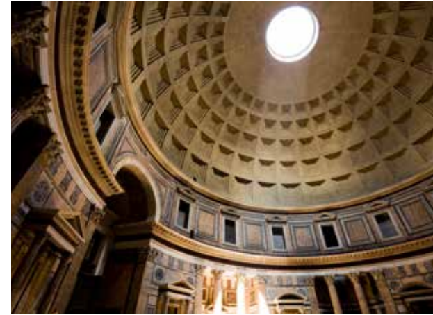
The rotunda of the Pantheon measures 43.5 metres in diameter which is exactly the maximum height of the dome, itself a perfect hemisphere. One of the most important features of the dome is the coffering which lightens the structural load and lightens the interior. Photo: Stock-Fotografie-ID:184291282, laughingmango
