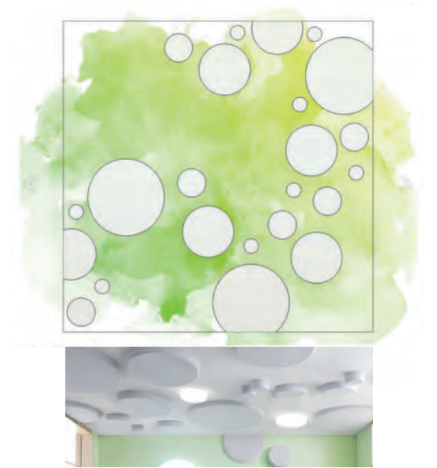
Sound insulation elements primarily serve to reduce noise levels. Mounted on the ceiling or wall, they fit naturally into the overall interior concept. Pictures: Wehrfritz
