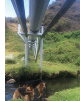
FIGURE 16. OIL PIPE FROM THE AMAZON. SOURCE: SELF TAKEN
