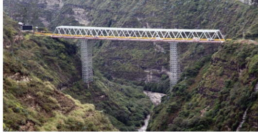
FIGURE 12. "EL CHICHE" BRIDGE BUILT AT THE END OF 1960S. SOURCE: HTTPS://NOTIMUNDO.COM.EC/SISMO-EN-QUITO-NO-REQUIRIO-ACTIVAR-EL-COE/
