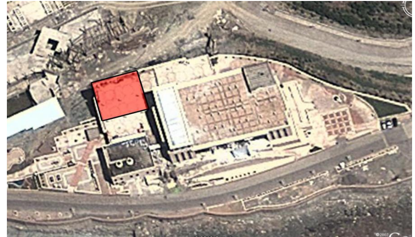
Image 08 : Membrane Structure Place On Building Terrace
