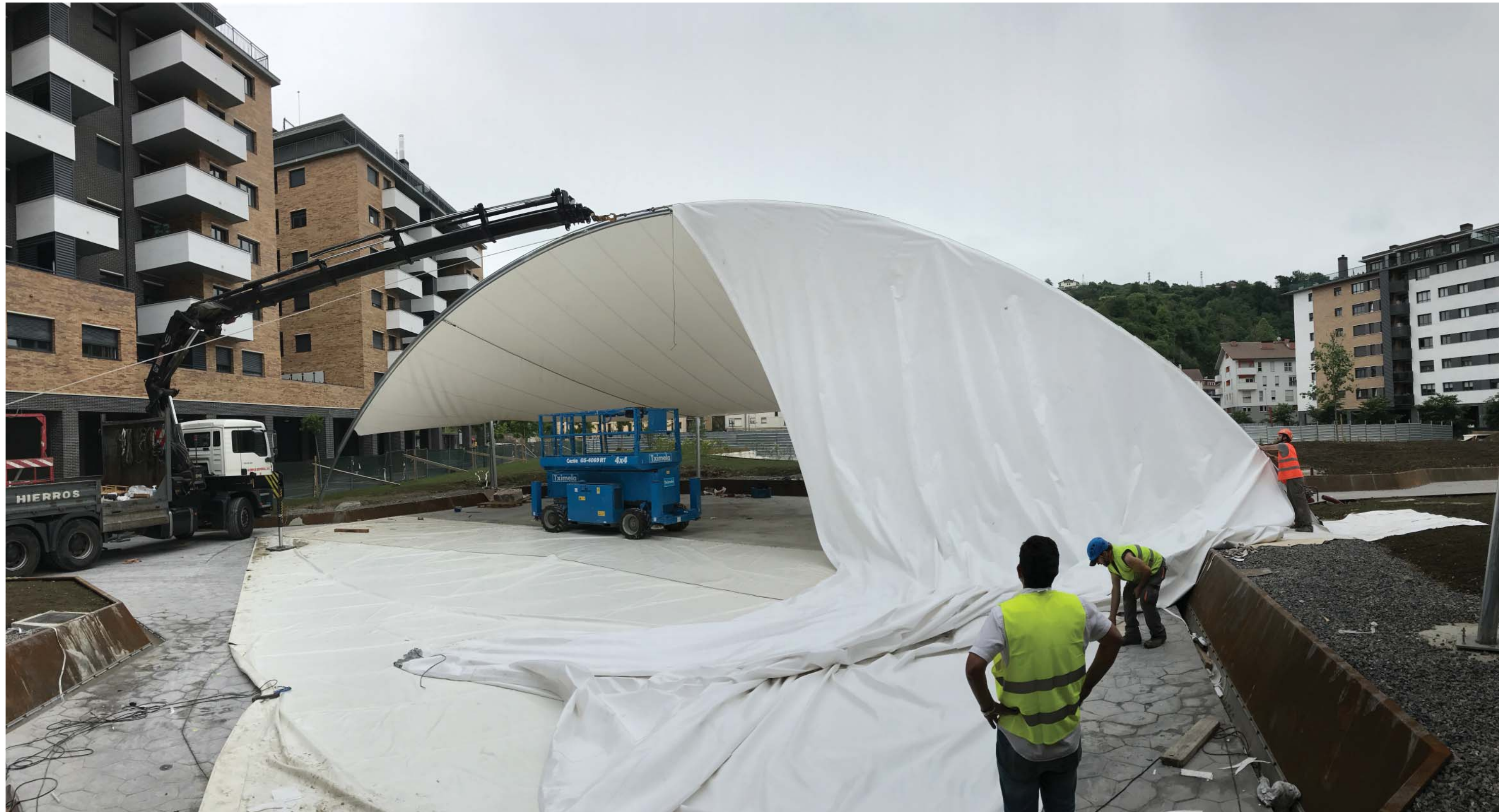
Membrane installation
