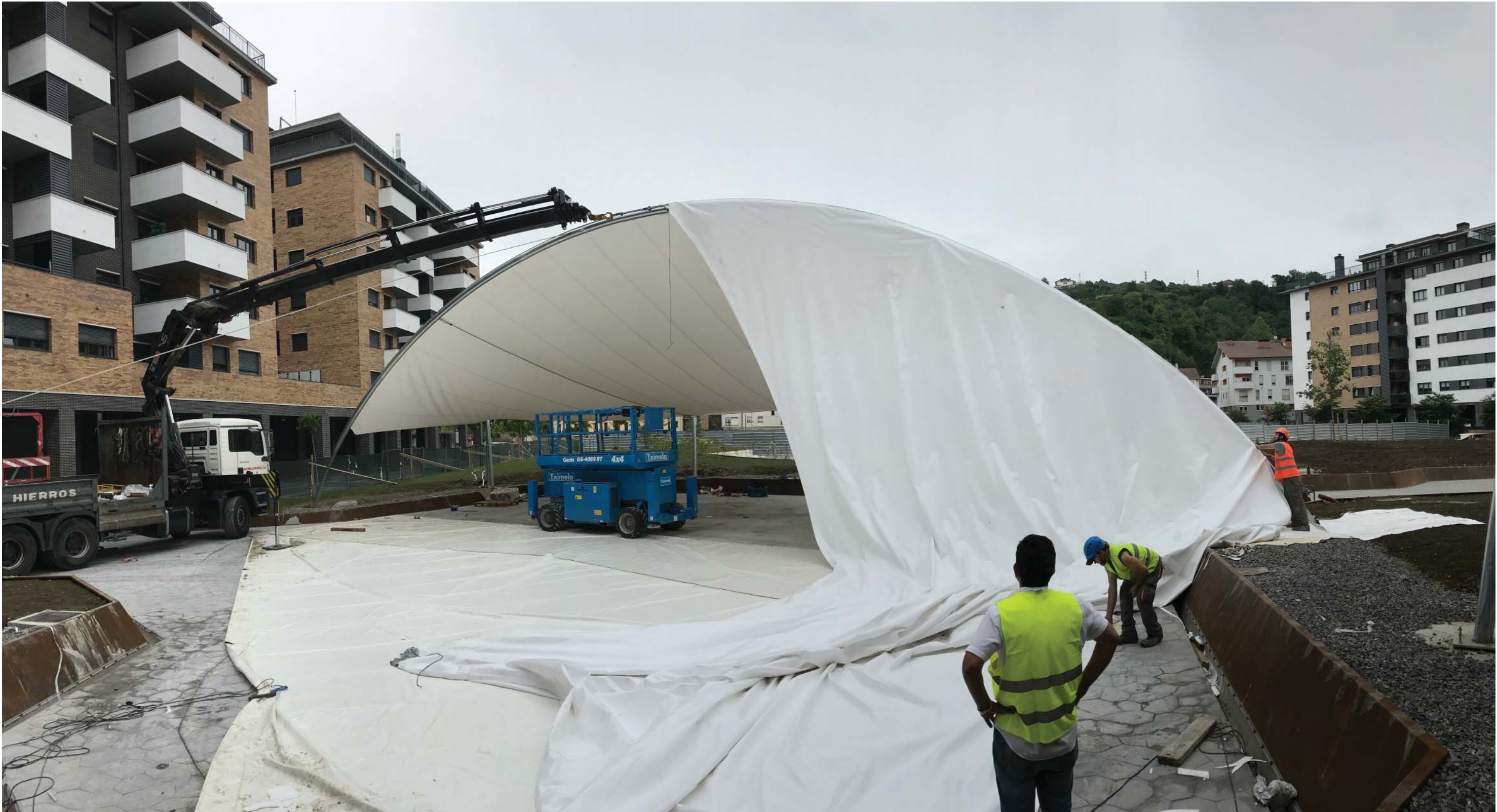
Membrane installation
