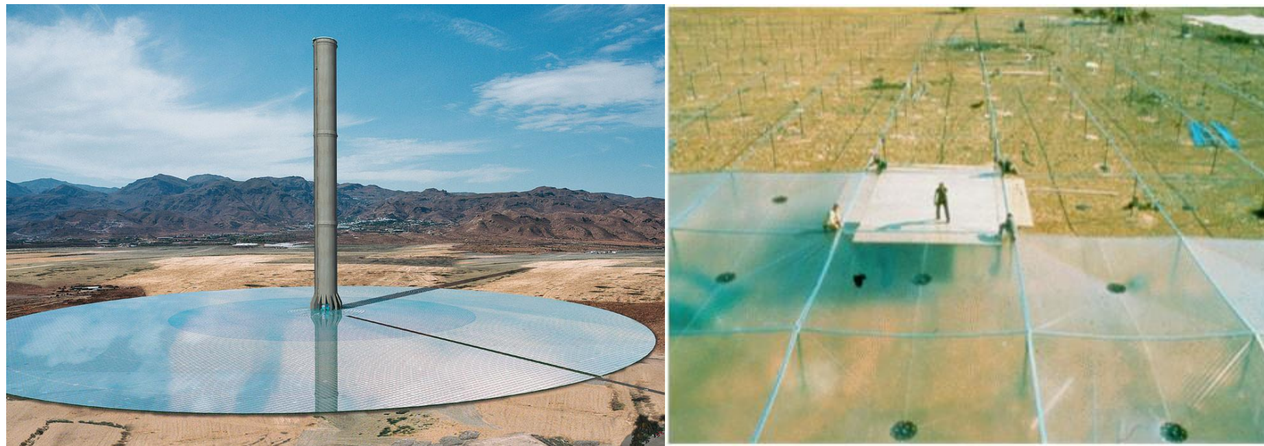
Figure 18 –Solar Updraft Tower (left) and ETFE film for solar updraft tower in Manzanara, Spain (right) (Copyright: Schlaich Bergermann und Partner)
