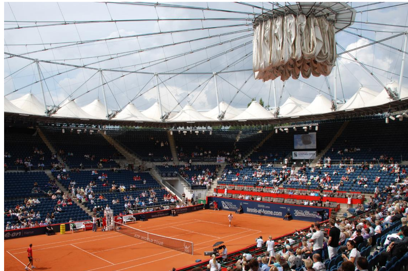
Figure 4 – Rothenbaum Tennis Court – Retractable Roof (Source: www.hamburg-web.de )
