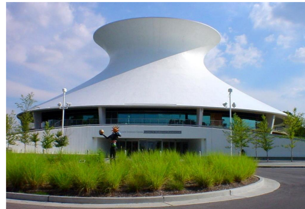
Figure 3.35 - Hyperboloid Shell of McDonnell Planetarium, by HOK Architects & A. Alper Structural. Engineer, St. Louis, MO, USA, 1963.
