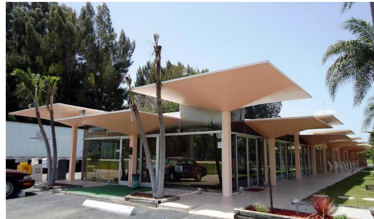
Figure 3.33 – Inverted Umbrellas, Warm Mineral Springs Inn Motel, by V. Lundy, Architect & D. Sawyer, Engineer, North Port, FL 1958.
