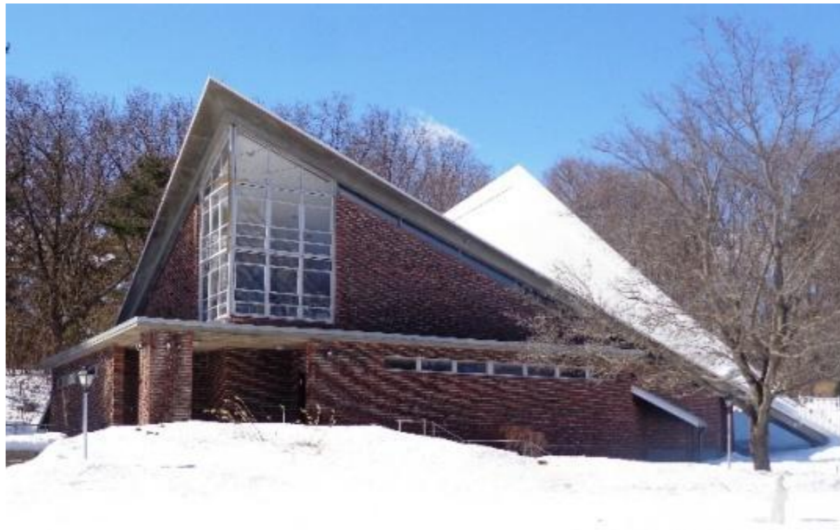
Figure 3.29 – St. Athanasius Church Hyperbolic Paraboloid Roof – Exterior Elevation Views of hyper concrete roof.
