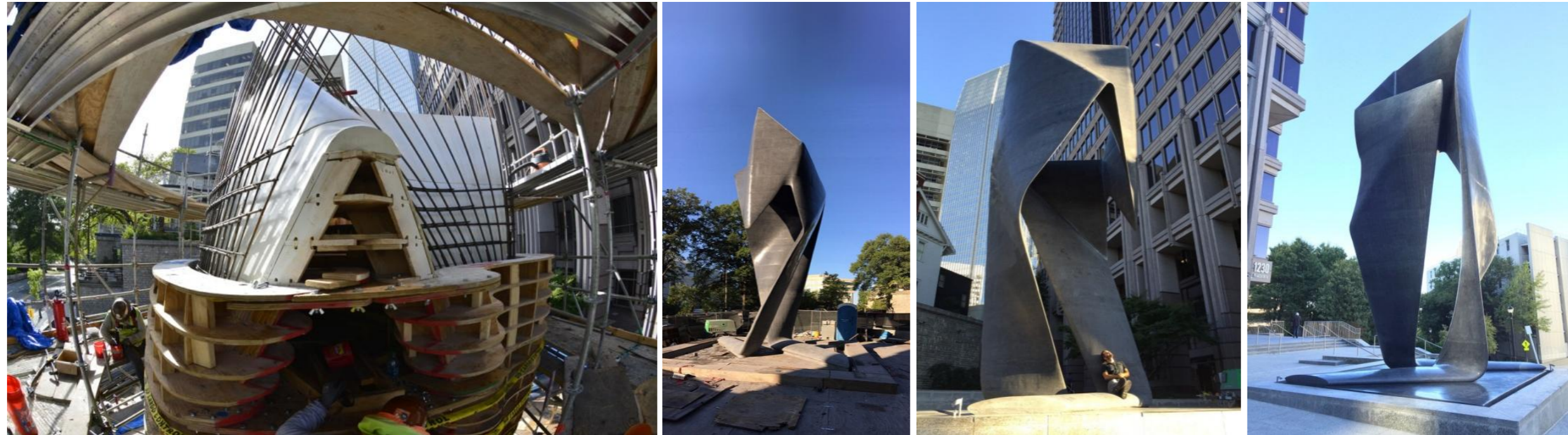
Figure 4.5 - The “Stealth“, Architectural Decorative Sculpture in Atlanta, Georgia, USA., Rebars, Formwork, and completed Sculpture.
