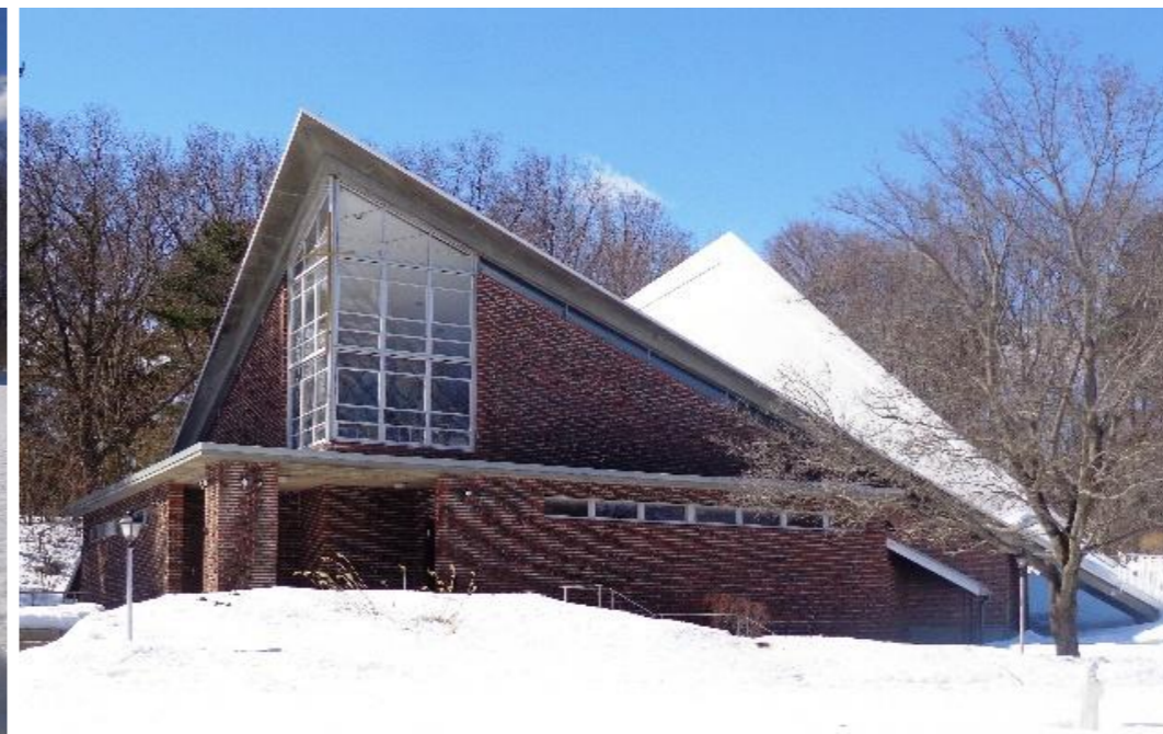
Figure 3.30 – St. Athanasius Church Hyperbolic Paraboloid Roof – Exterior Front and Side Elevation Views of hyper concrete roof.
