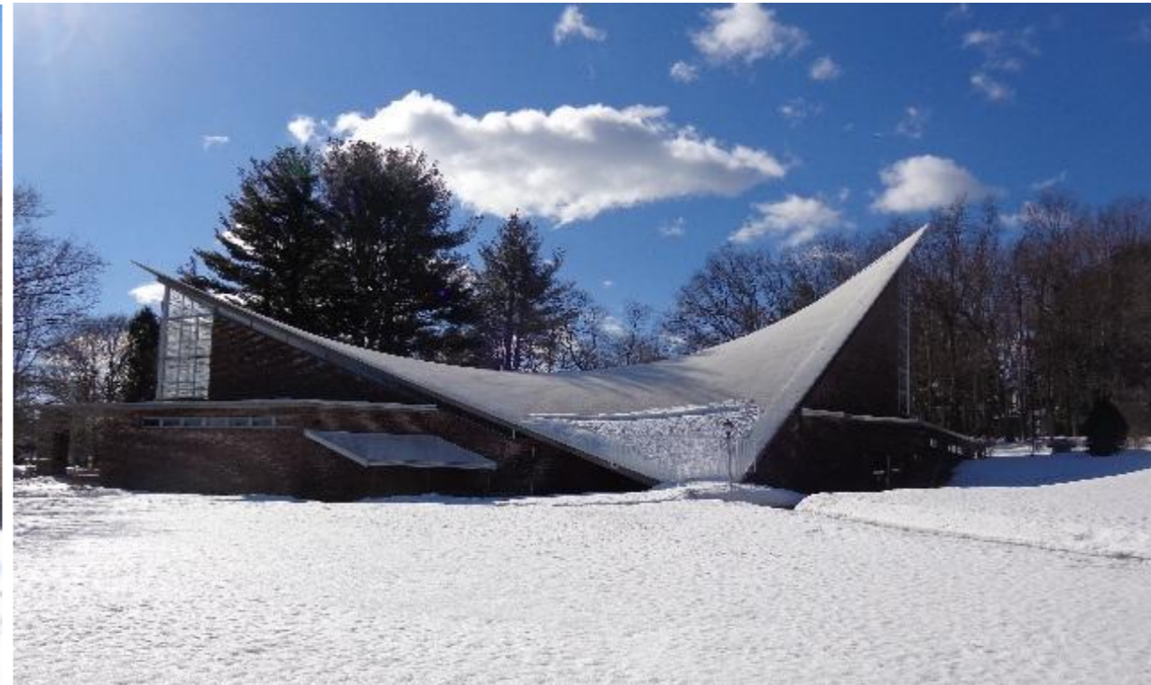
Figure 3.29 – St. Athanasius Church Hyperbolic Paraboloid Roof – Exterior Elevation Views of hyper concrete roof.
