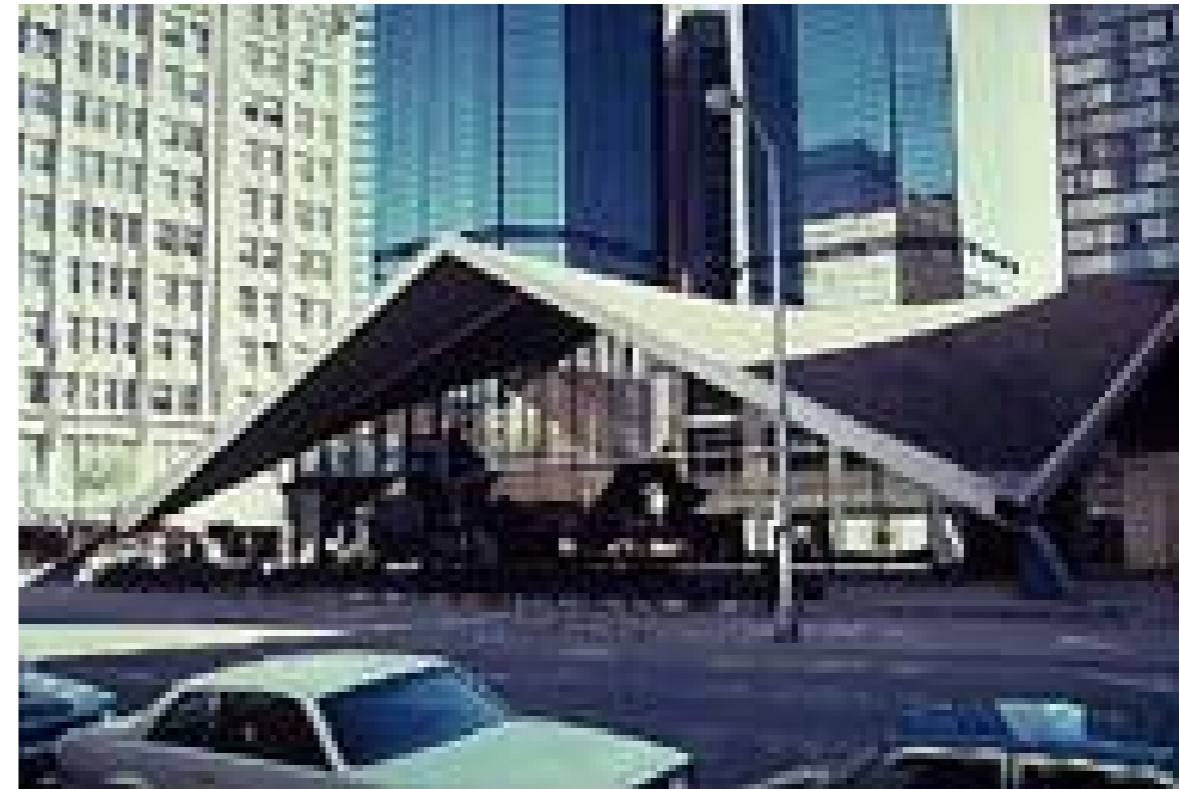
Denver Courthouse Square, Denver, CO, 1958 – by: A. Tedesko “Demolished in 1996”
