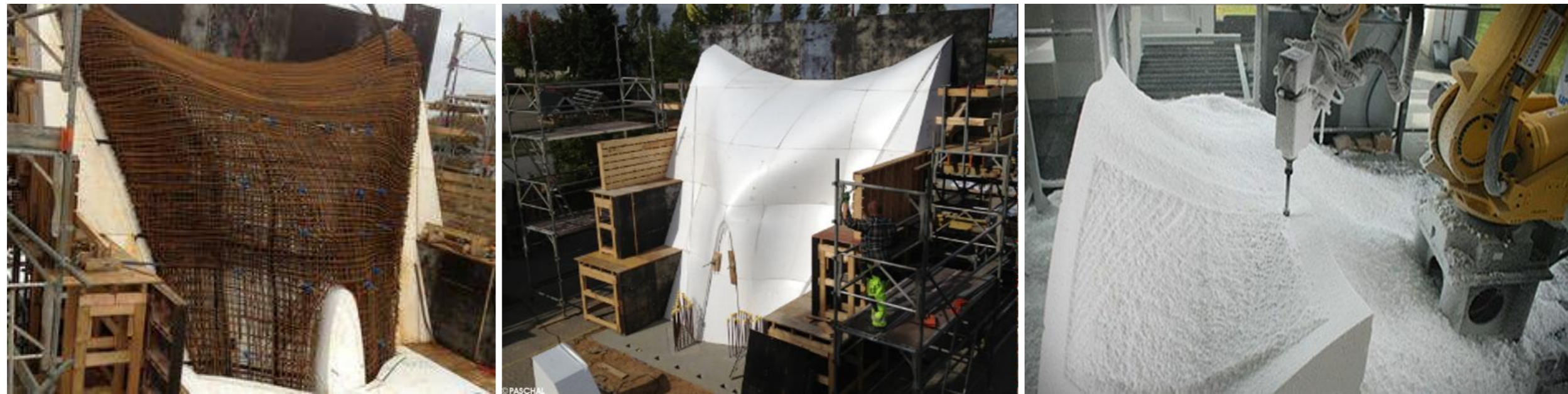
Figure 4.4 - The TailorCrete Project, “Demonstrator“, Danish Technological Institute (DTI), Steel Rebars and Robotic Generated Formwork.
