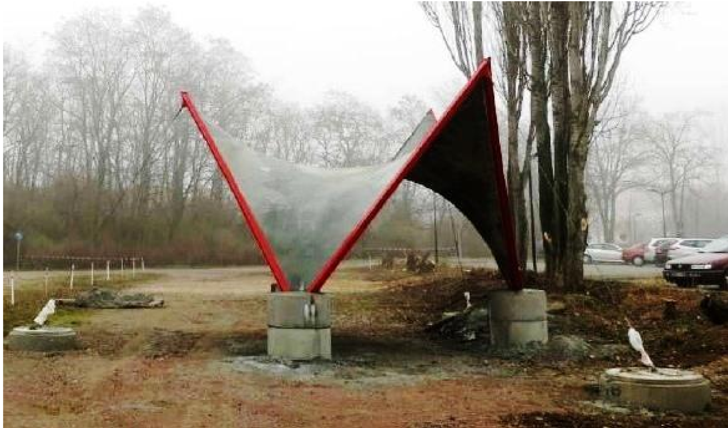
Figure 5.38 – View of completed Membrane-Concrete Shell Structure, edge beams, cables, and concrete bases right after completed construction.
