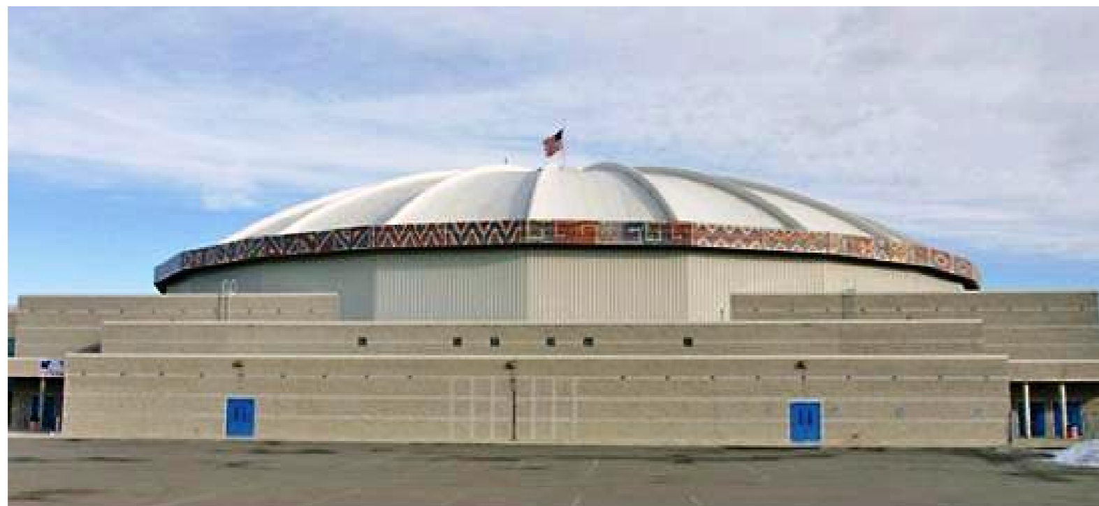
Figure 3.23 - Loofburrow Architects; J. Christiansen Engineers – 1990; Yakima, WA – USA; R = 248 ft., t = 3.75'' – R/t = 794 .
