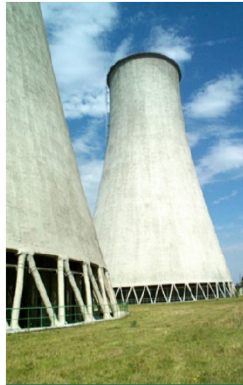
Cooling Towers, Europe
