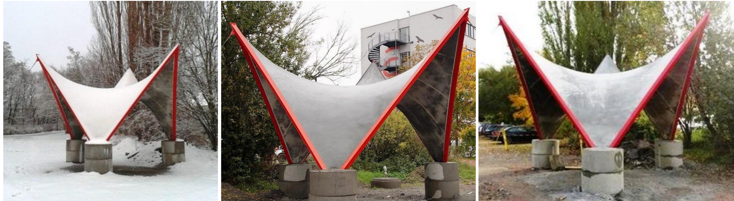
Figure 4.20 – Pictures of completed membrane-concrete shell prototype after hardening of shotcrete and finished shell surface.
