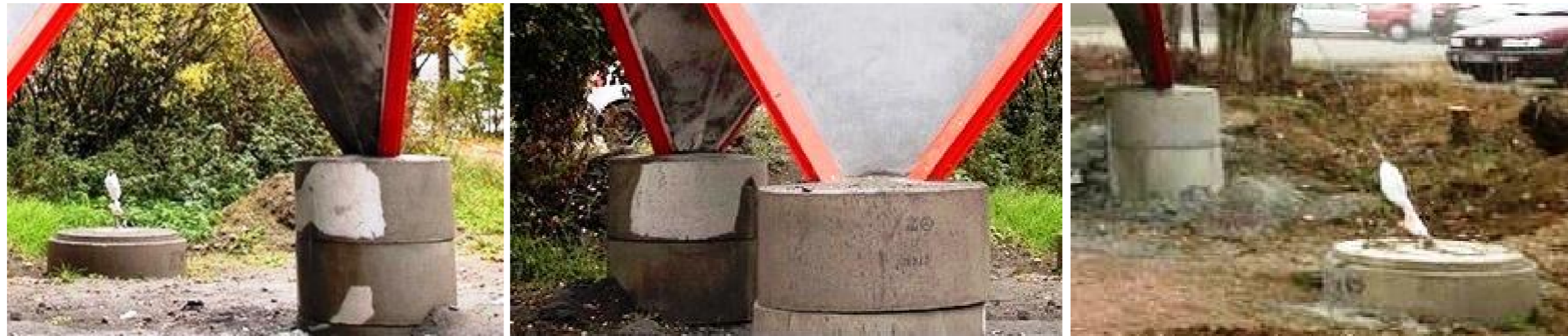
Figure 4.18 - Constructed Tensioned Membrane-Concrete Shell, Steel Frame and Tie-down Cable Connection Details to Concrete Bases.
