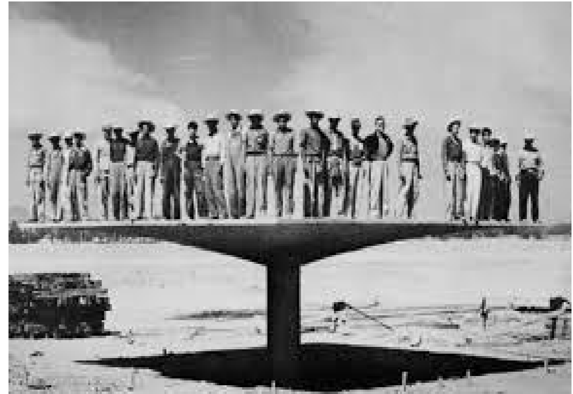
Figure 3.48 – Felix Candela thin reinforced concrete inverted umbrella shell project built in Mexico, Formwork and Elevation View.
