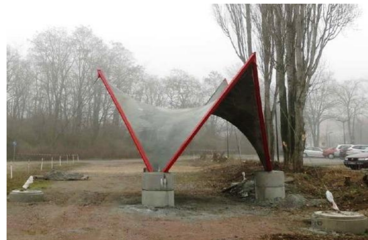
b) Constructed Membrane-Concrete Shell Prototype – March 2014
