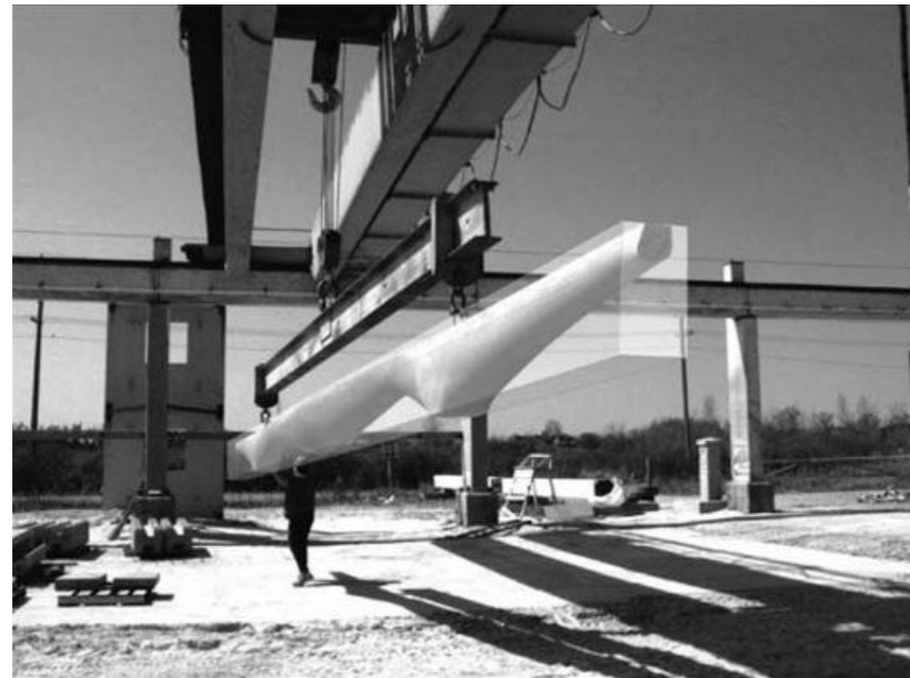
Figure 4.1 – Fabric Formed Beams, by Mark West
