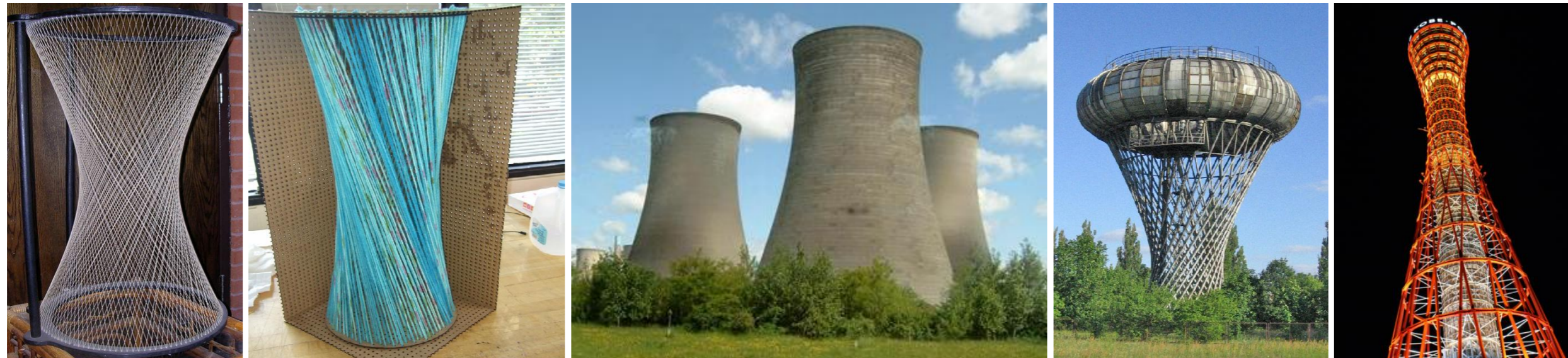
Figure 1.12 – Physical Models of Hyperboloids and different types of as-built Hyperboloid structures around the world.
