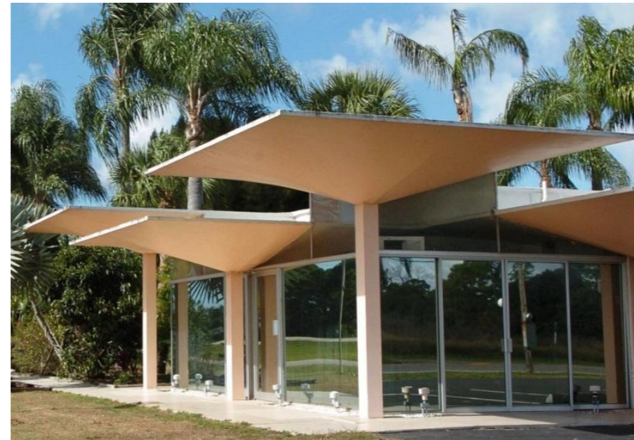
Warm Mineral Springs Inn Motel, North Port, FL, 1958– by Candela, Today Demolished.
