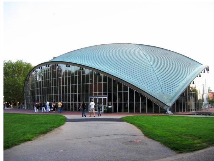
Figure 3.21 - Eero Saarinen & Associates, Architects – Ammann & Whitney – 1955; Cambridge, MA – USA; R = 112 \text{ ft.} , t = 3.5'' – R/t = 384 .
