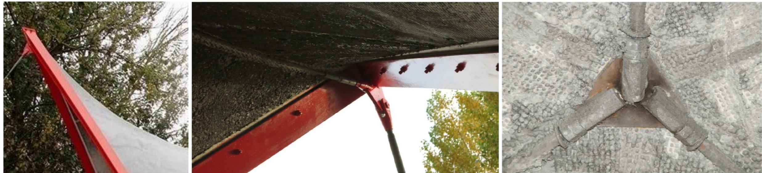
Figure 4.17 – Constructed Tensioned Membrane-Concrete Shell, Steel Frame and Cable Connection Details to Steel Frame.
