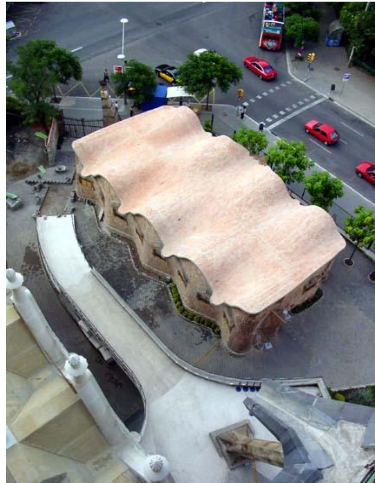
Figure 1.15 – Church of Christ the Worker Conoidal Brickwork Walls – Conoidal Brick Roof of Gaudi’s School of Sagrada Familia in Spain.
