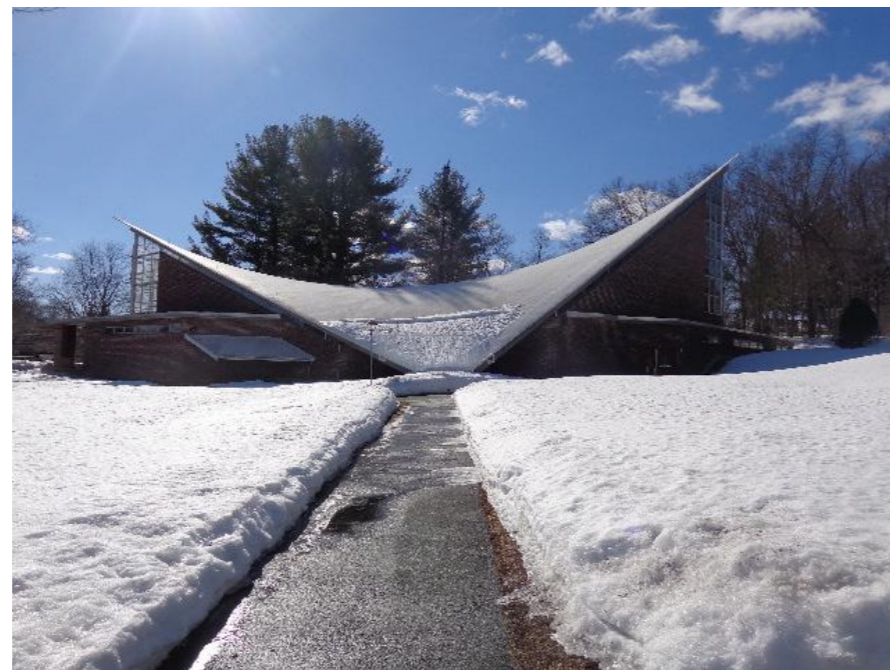
Figure 3.30 – St. Athanasius Church Hyperbolic Paraboloid Roof – Exterior Front and Side Elevation Views of hyper concrete roof.
