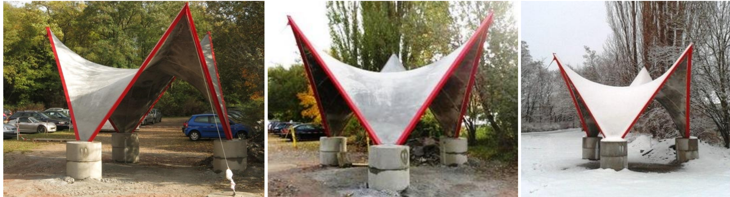
Figure 5.3 – Pictures of the completed IMS Membrane-Concrete Shell Prototype with the entire shotcrete shell surface installed.
