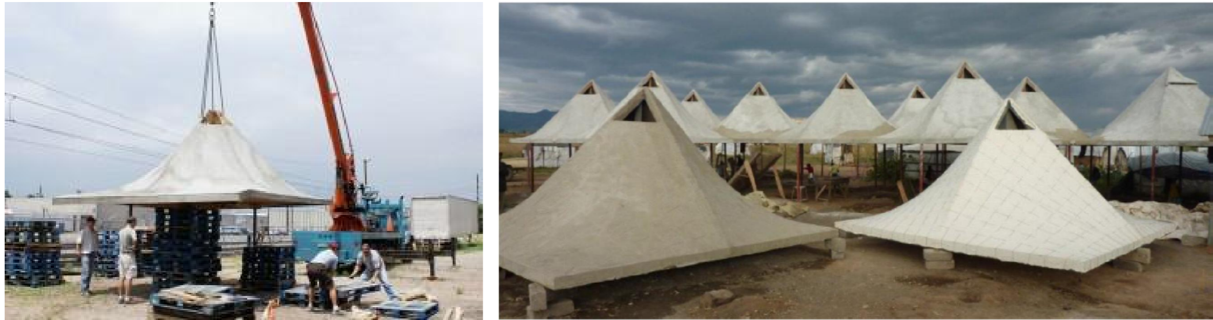
Figure 4.8 – Thin Shell Composite Hyperbolic Paraboloid Roof, TSC Hypar, built by TSC Global LLC Company for African Nations.
