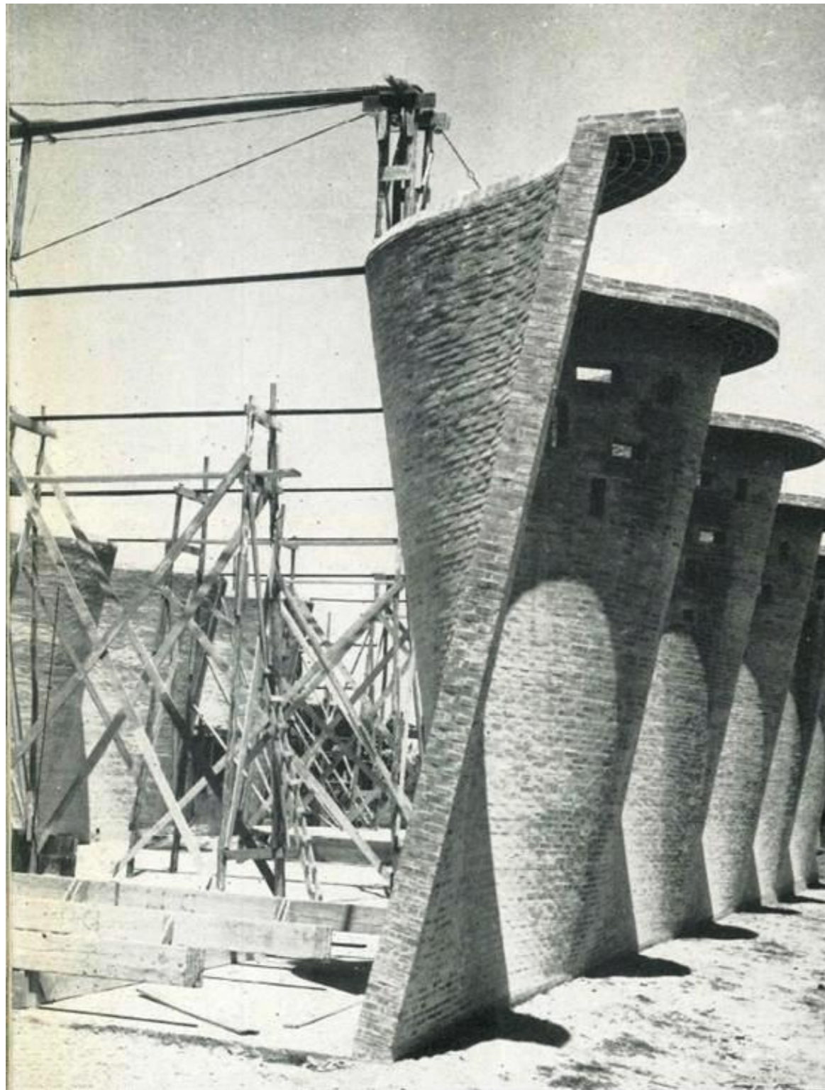
Figure 1.15 – Church of Christ the Worker Conoidal Brickwork Walls – Conoidal Brick Roof of Gaudi’s School of Sagrada Familia in Spain.
