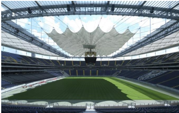
Figure 9: Commerzbank-Arena Frankfurt toldo shading in semi retracted position, Frankfurt, Germany (Schlaich Bergermann Partner, 2006)
