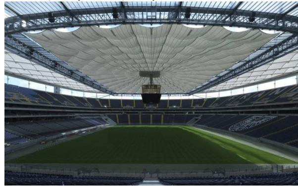
Figure 10: Commerzbank-Arena Frankfurt in almost deployed position, Frankfurt, Germany (Schlaich Bergermann Partner, 2006)
