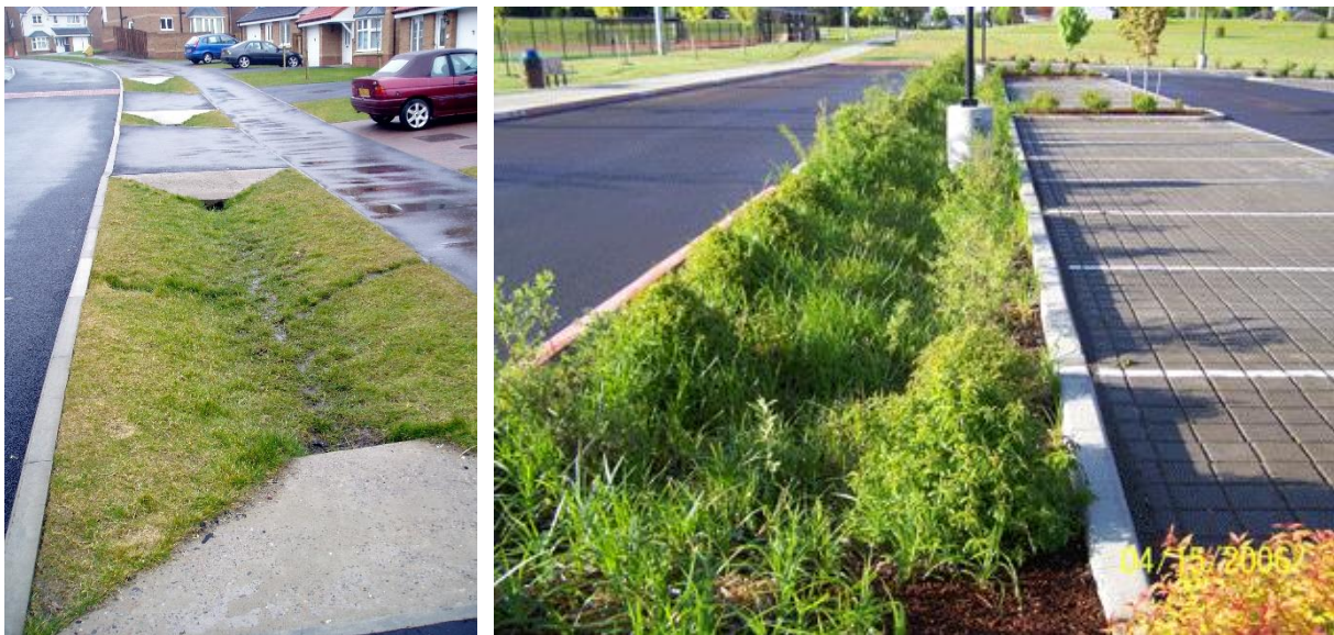
Figure 2.12: Swale on left, Bio Retention Swale on Right ( https://www.susdrain.org/delivering-suds/using-suds/suds-components/swales-and-conveyance-channels/swales.html , 12.10.20, https://catalog.extension.oregon-state.edu/em9209/html,12.10.20 )
