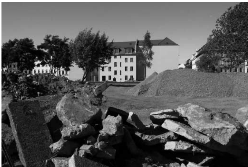
Figure 2 ■ Large-scale demolition of densely built-up housing structures in inner parts of the Wilhelminian city: new open spaces for experimental design of recreational green infrastructure? (Photo: D. Haase)
