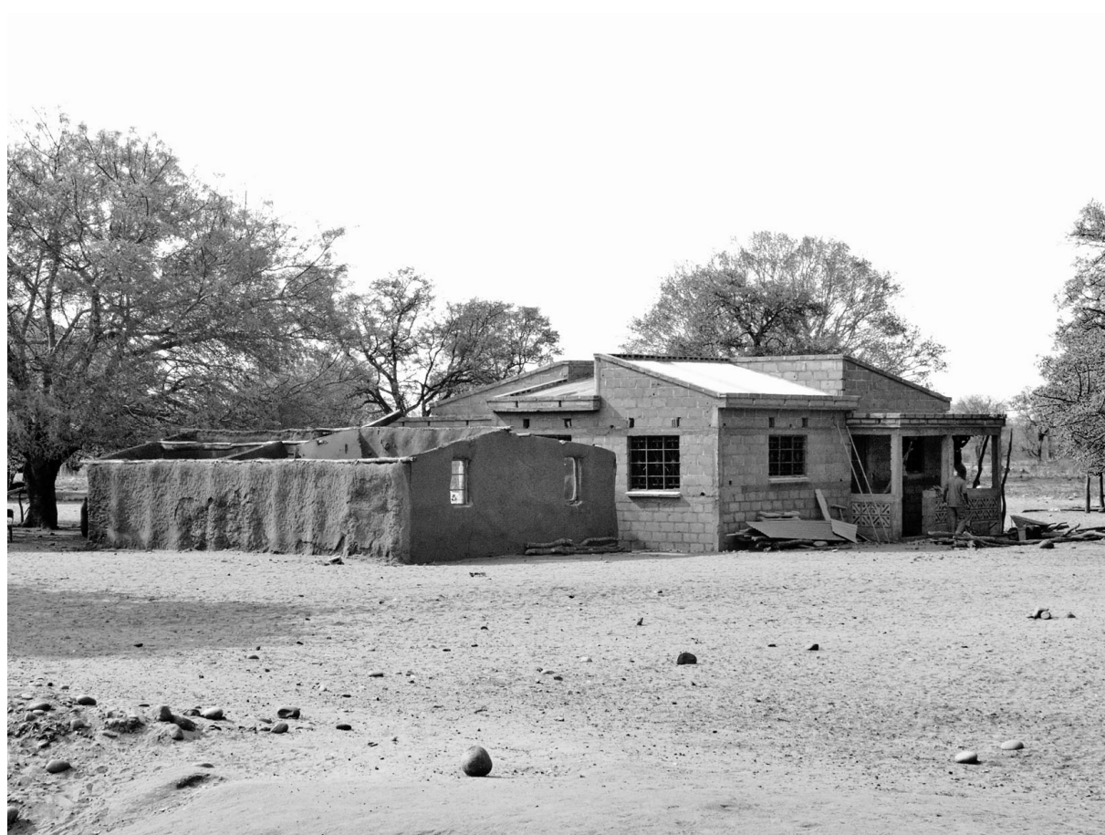
Figure 56 - Brick house being built close to old house in Canhane (photograph by the author, March 28, 2008).
