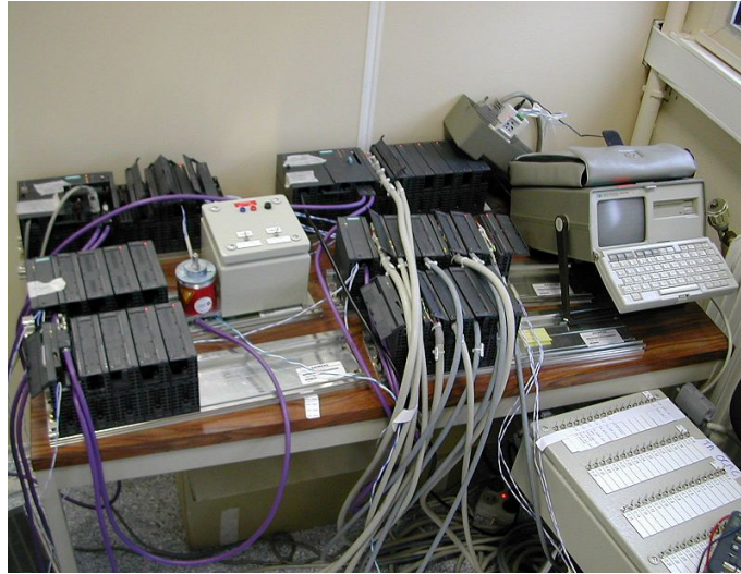
Figure 2.4: An example of PLC.
