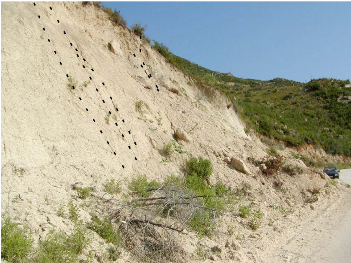
Fig. 3.6: Slope failure within marly sands at a location where the slope is cut and disturbed by fault planes (the revealed fault traces are shown by dashed lines). The geometry of the fault planes and the failure plane are irrelevant to each other.
