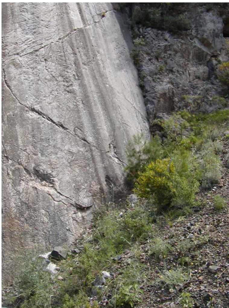
Fig. 4.13: Overview of the location on the eastern segment of the Shinos fault which was selected for the installation of the second monitoring site. In the background, the hanging wall (right hand side in the photograph) as well as the footwall (on the left) consist of Triassic limestone.
