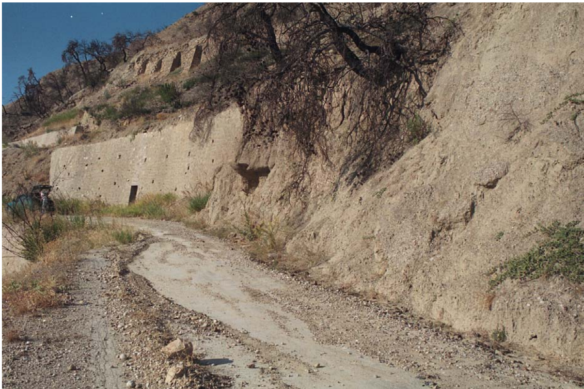
Fig. 3.5: Extensive mass movements in sandy marls and intercalating loose conglomerates with loamy matrix after deforestation (fire) which allowed slope instability to initiate in areas where slope supporting measures were formerly not necessary.
