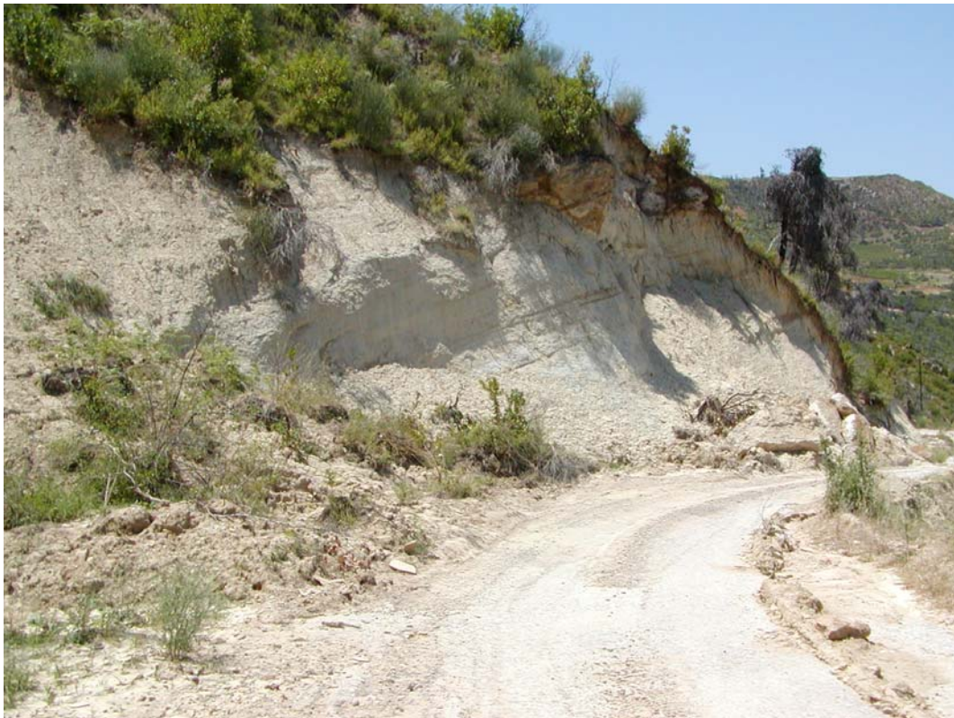
Fig. 3.3: A slope failure within sandy marls disrupting a road and triggered by rainfall. Deformation on the road surface implies that the instability extends also below the road i.e. the entire slope is moving.
