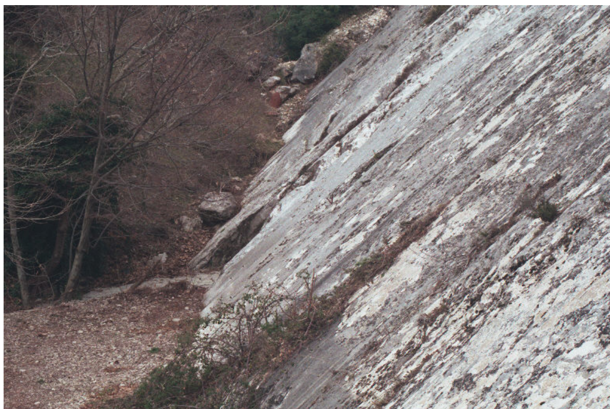
Fig.4.9: The selected location along the Pisia fault escarpment for the first installation of the TM71 and the Bragg Grating Extensometer. In the background, the gully where the instrument were installed is visible. On the right (south) the fault plane on Triassic limestone (footwall) is visible whereas on the left (north) the hanging wall consists of pleistocenic material.
