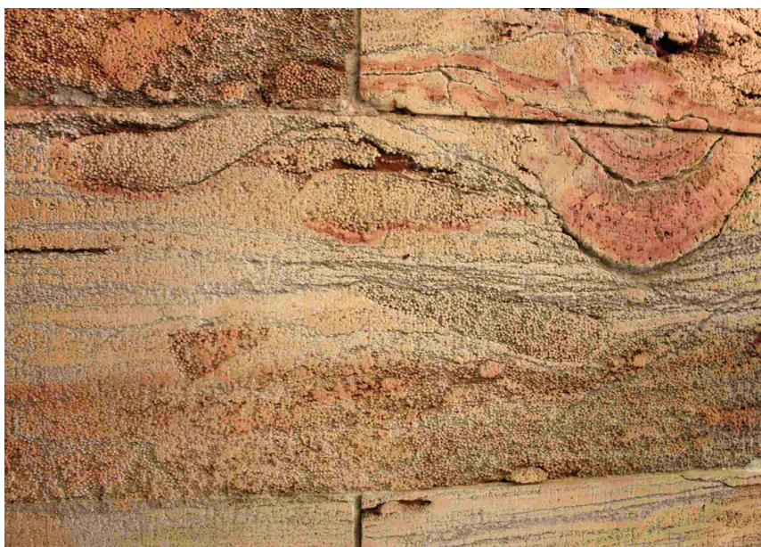
Fig. 4 Freestones of the Old Town Hall: Oolites and a stromatolite dome. The freestone block has been placed upside down. Thickness of the freestone is about 30 cm.
