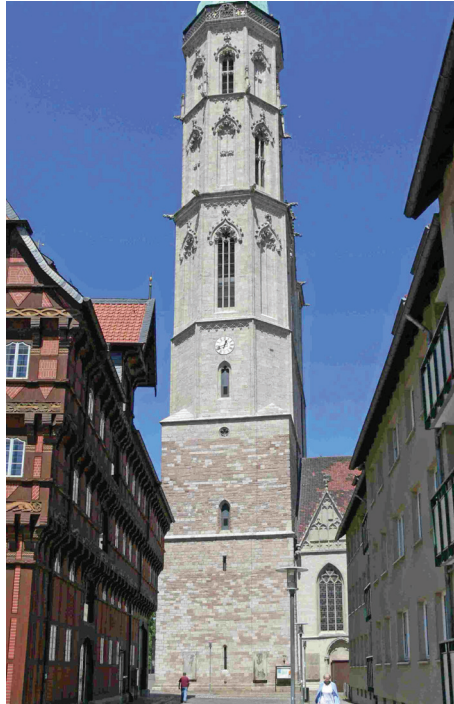
Fig. 2 The spire of the Andreas Church in Braunschweig. The lower part is built mostly of red and white rogenstein whereas the upper part consists of white Muschelkalk freestones.
