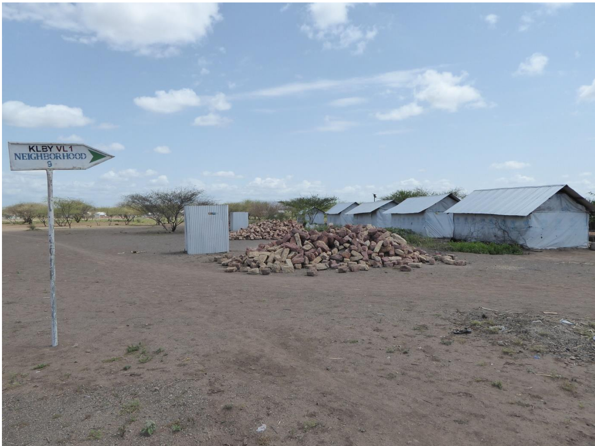
Figure 10. Shelters in Kalobeyei awaiting construction.
