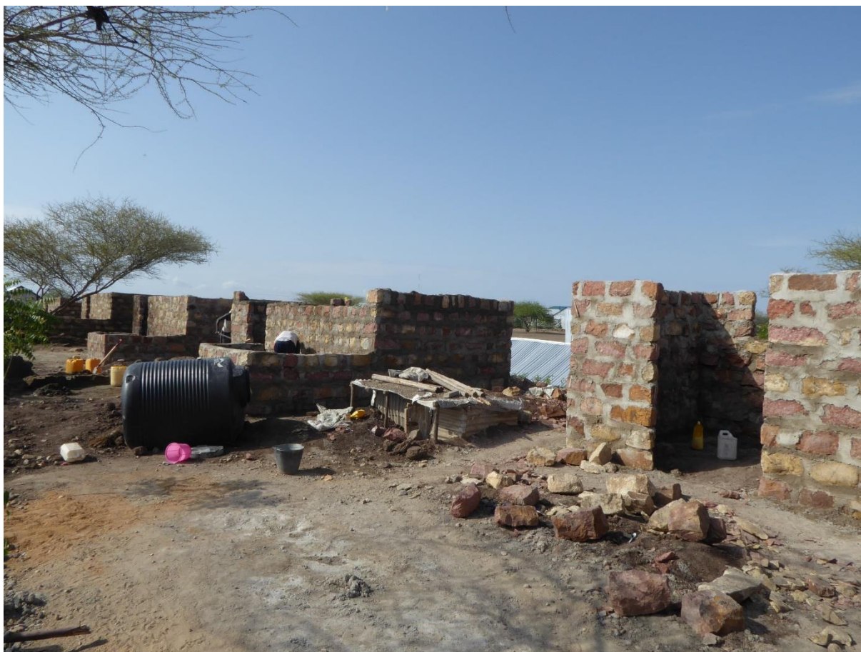
Figure 11. The construction of permanent shelters, Kalobeyei.
